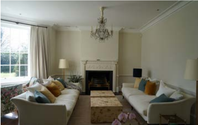
Non-historic fireplace in south wall
