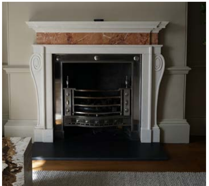
Non-historic fireplace in north wall
