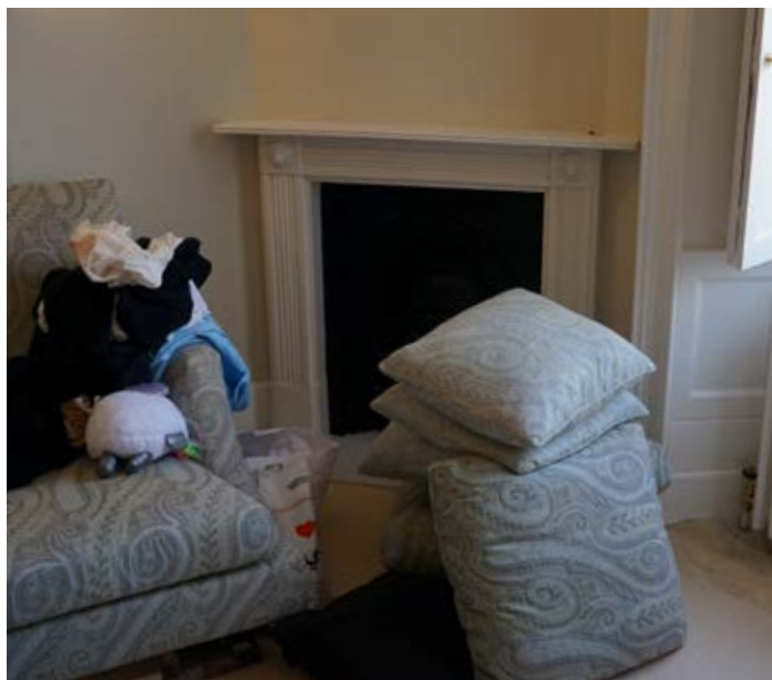
Non-historic fireplace in south-west corner of dressing room
