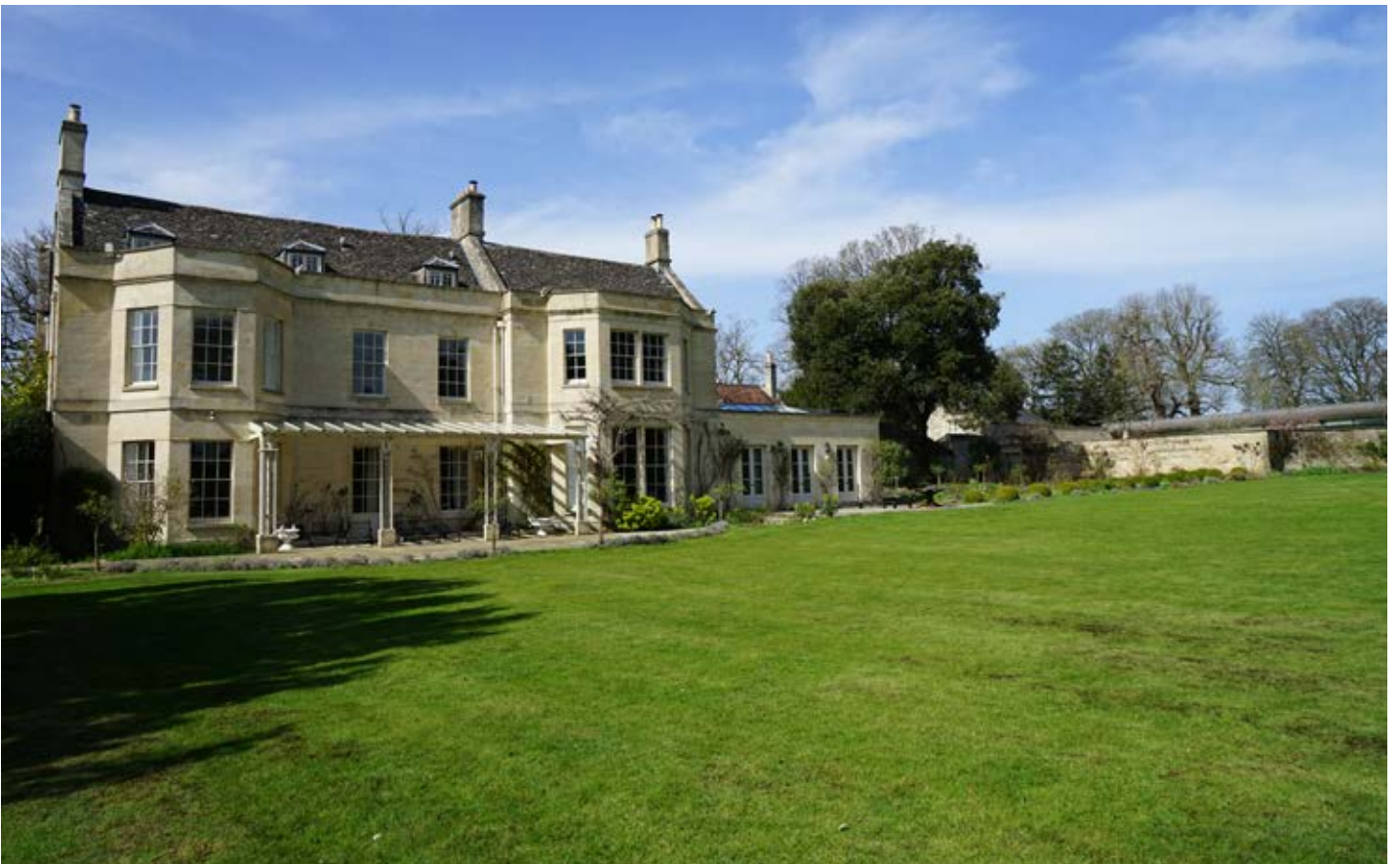
East elevation; John Cary's mid-18th century 'garden front'
