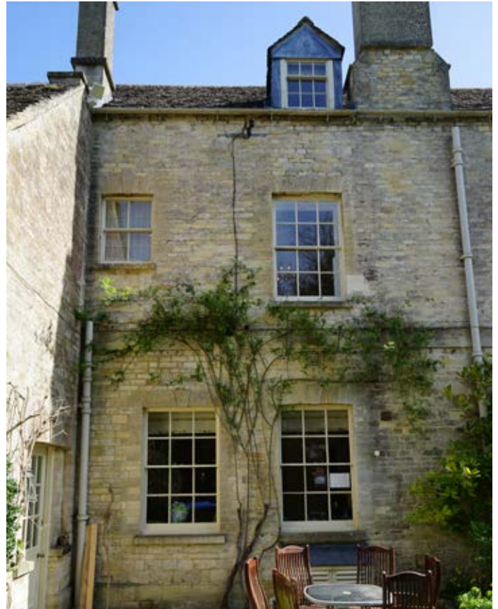
External view of terrace and west-side kitchen windows
