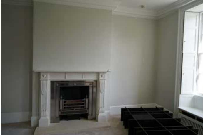
North wall of current master living room
