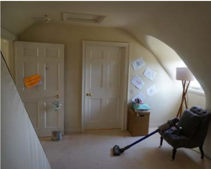
Current doorway to hall (left-hand side) and doorway to ensuite
