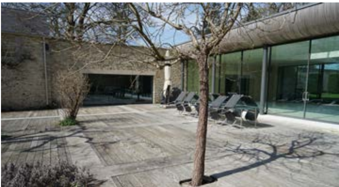
East elevation of pool house, to north side of walled garden
