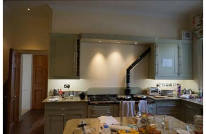
South wall of kitchen adjoining morning room, non-historic partition. The flue from the aga diverts through the wall, and no fireplace or chimney would be affected by the partition's removal
