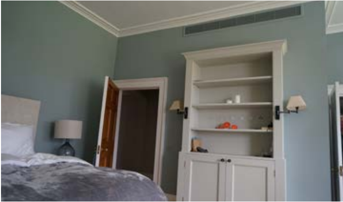
Non-historic partition, with door to hallway on left-hand side
