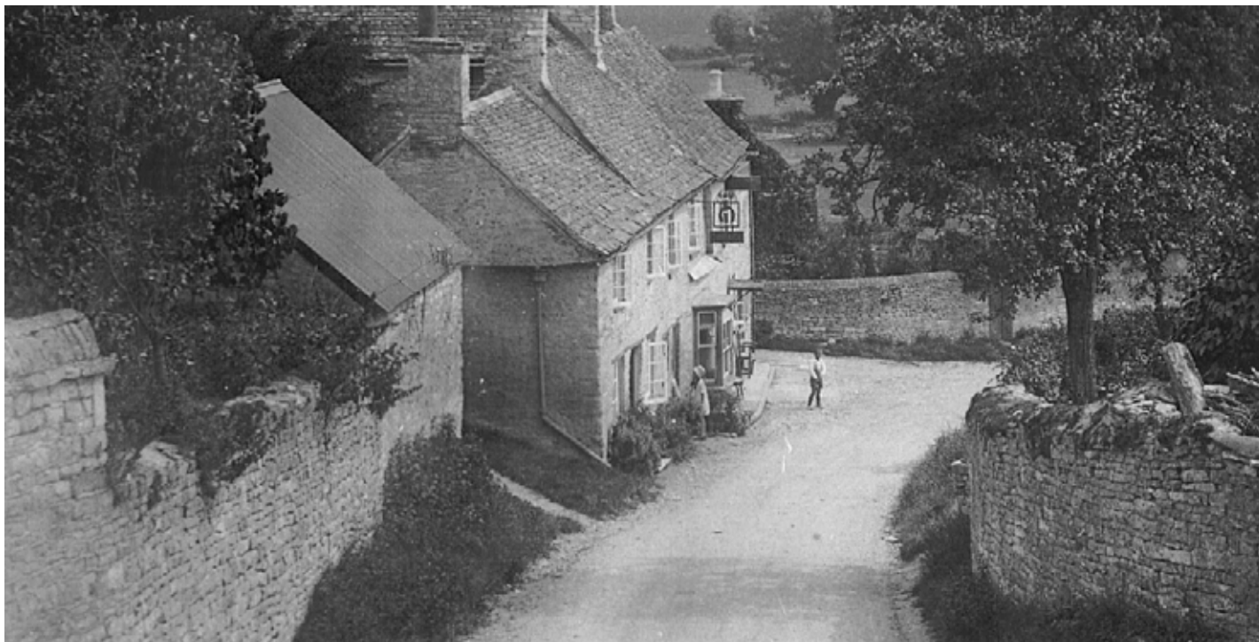
View Horseshoe Lane showing stone rubble walls and stone slate roof with diminish courses.
