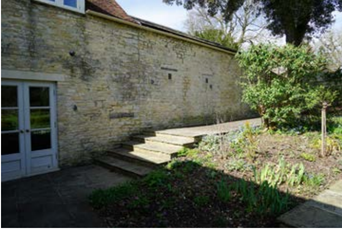
External view of stable block east wall
