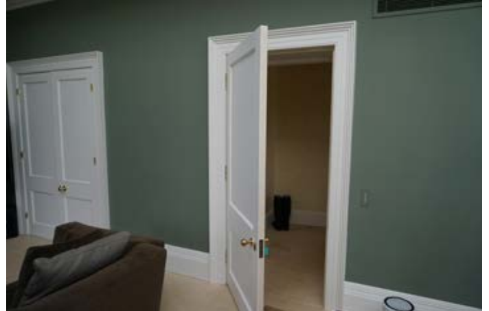
West door of garden room leading to back hall (right-hand side), and door to boiler room (left-hand side)
