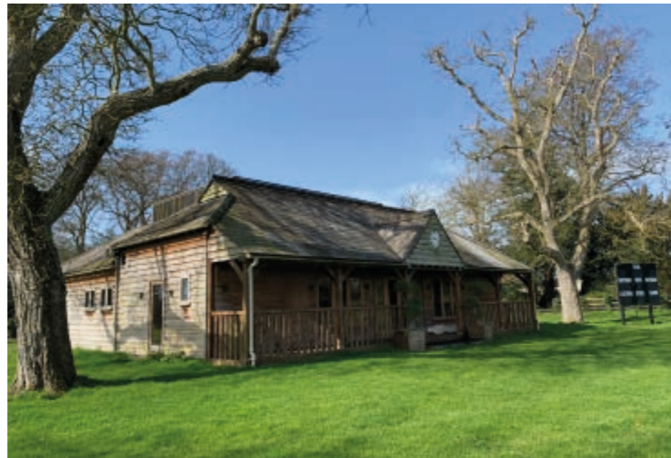
5 view towards cricket pavilion
