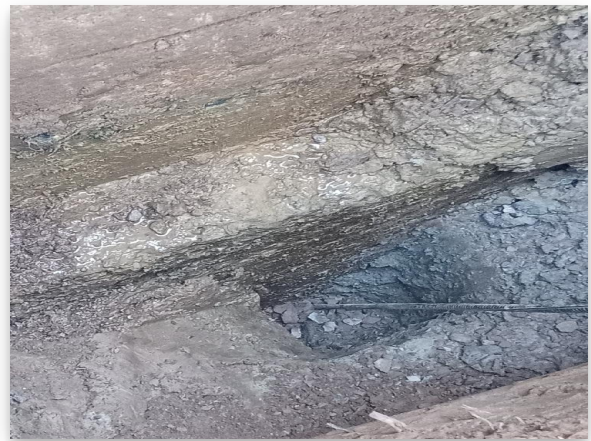
Fig 1.2: Trial Hole 2 Footing
