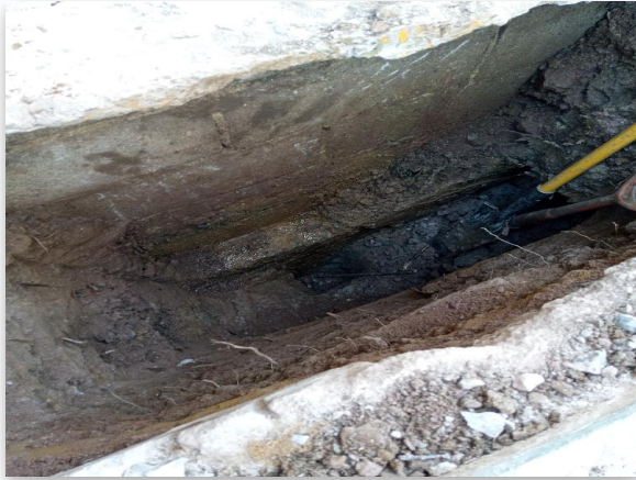
Fig 2.1: Trial Hole Open
