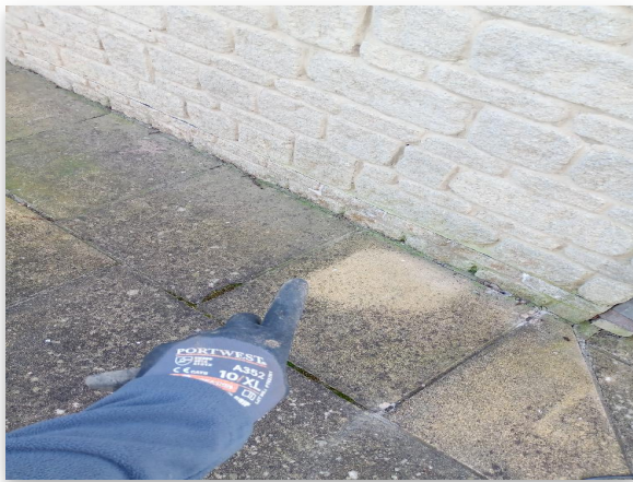
Fig 1.1: Trial Hole 2 Location
