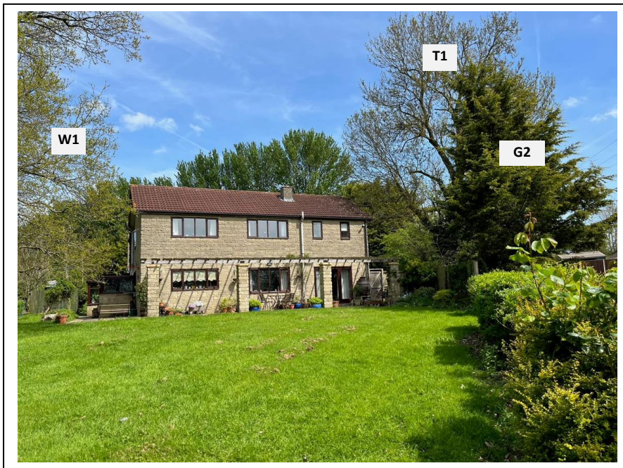
View of rear elevation, W1, T1 and G2
