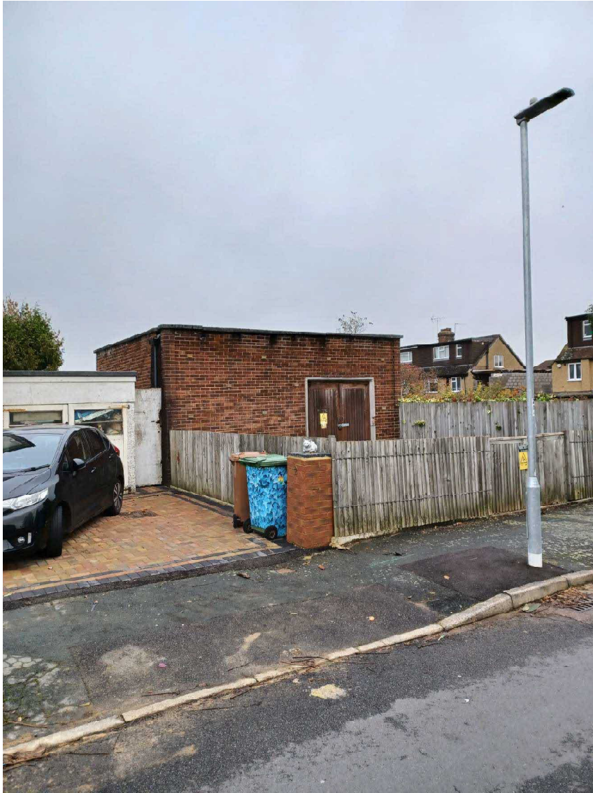
Part front elevation and the adjacent sub-station
