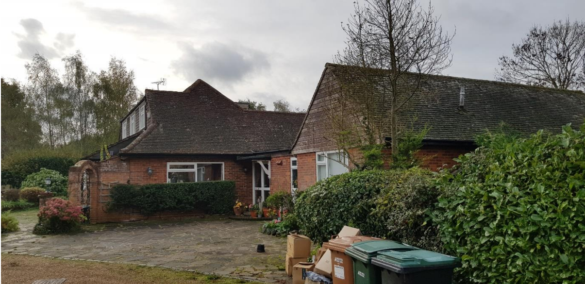
Fig 4 View of side of existing house
