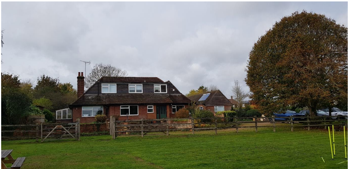
Fig 3 View of front of existing house
