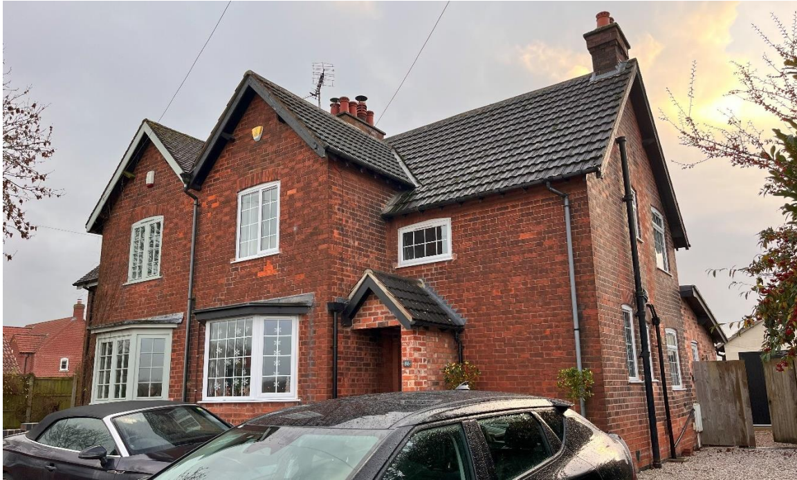
Photograph 1: 86 Caythorpe Road, taken from the north-west, showing the two-storey dwelling and its L-shaped footprint, along with the interlocking roof tile feature and exposed timbers on the gables and eaves.
