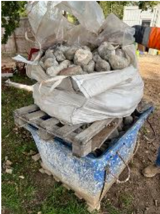
3.3 Fig 3 - Flints Salvaged for South Facing elevation
