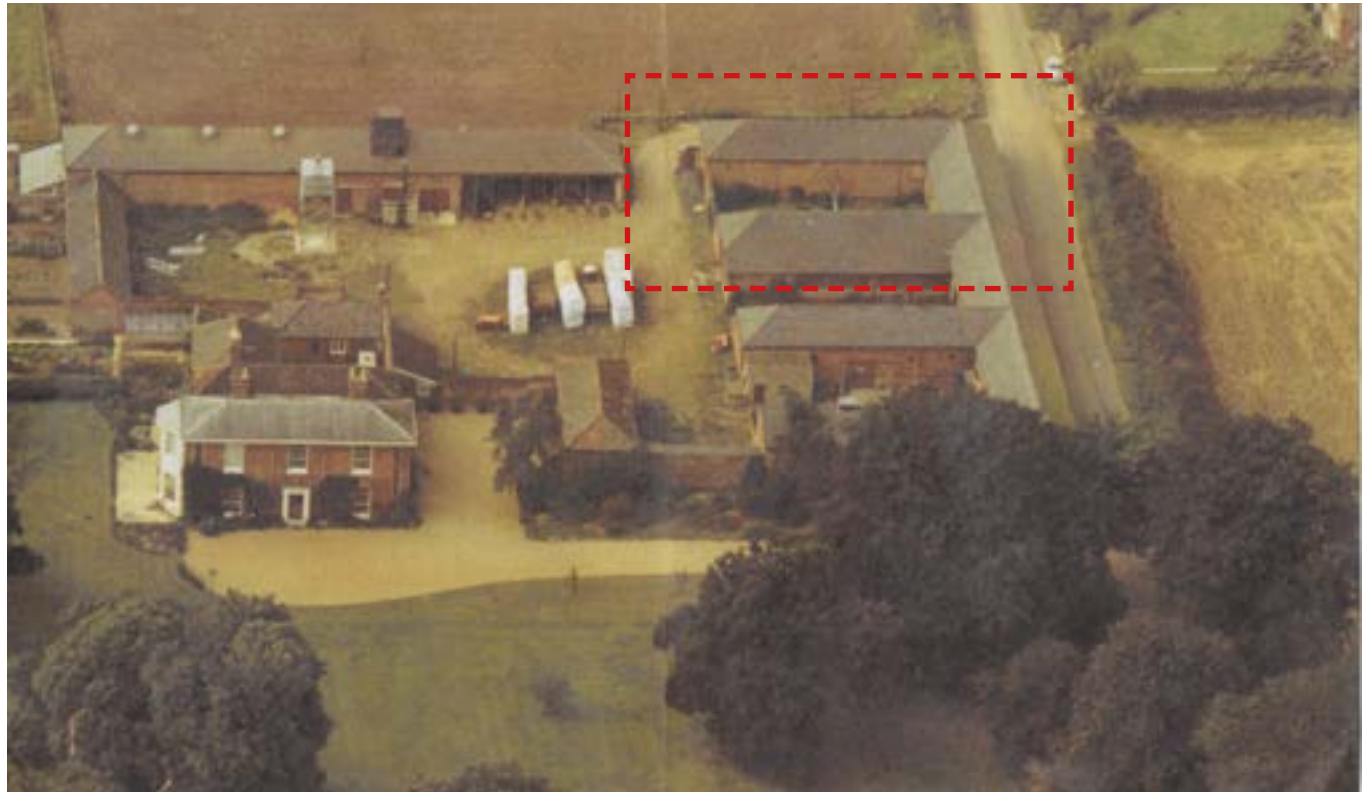
Figure 1: Aerial photo taken pre-conversion September 1971. The Manor House is bottom left of the picture. The application site is highlighted with a red dotted box.
