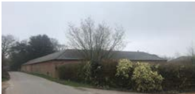
View looking south east from main road. No changes proposed.
