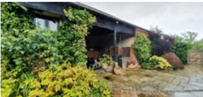
View of west facing inner courtyard elevation: no changes are proposed to these openings but the windows are proposed to be replaced. And a tools & logs store is being proposed to the back of the cart shed.
