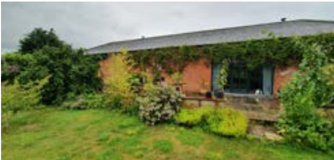
View of west facing elevation: no changes are proposed to these openings but the windows are proposed to be replaced.
