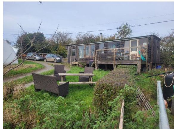
P4: Site: viewed from the SE corner, looking N
