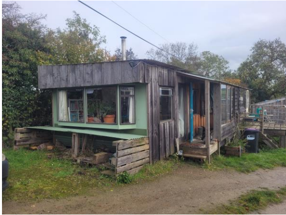
P1: W (end) + S (side) elevations: looking ENE
