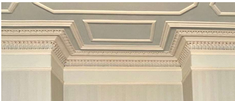
Figure 10 – Cornice and Picture Rail in Lounge
