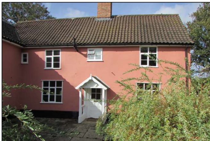
Figure 6 - South-east elevation of no.2 The Lodge.
