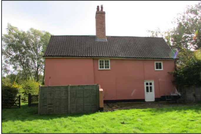
Figure 10 - Rear/ west elevation of no. 2.
