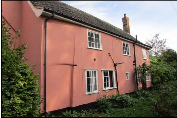
Figure 13 - Rear elevation of no. 1.
