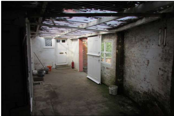
Figure 18 - Reverse view within the yard.
