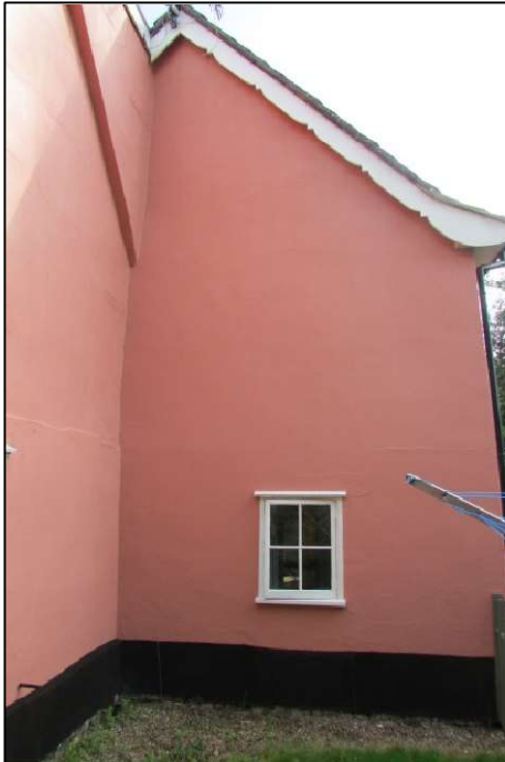
Figure 15 – Later link/west gable of no. 1, adjoining the above.
