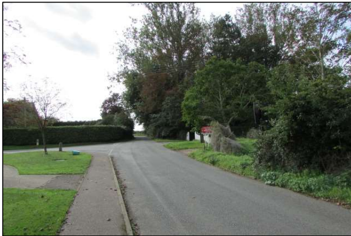
Figure 31 - View South along Norton Road, including the site entrance.
