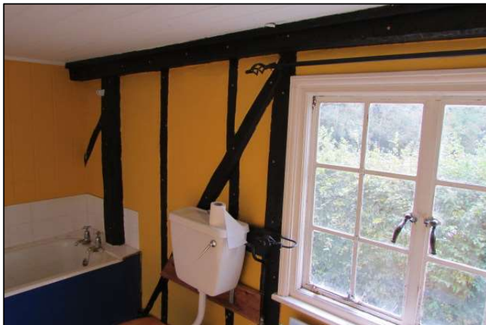
Figure 21 - Main bathroom to no. 1.
