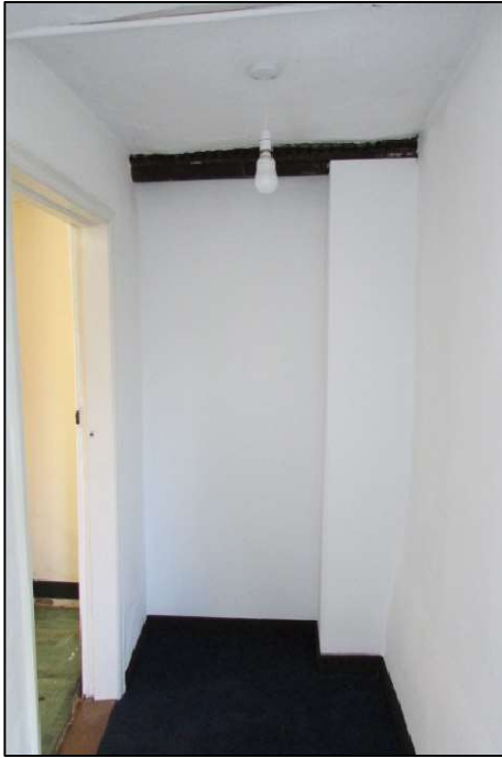
Figure 20 - as above viewed from within no. 1.
