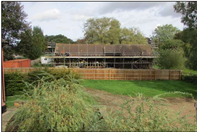
Figure 34 - as above with the barn behind.
