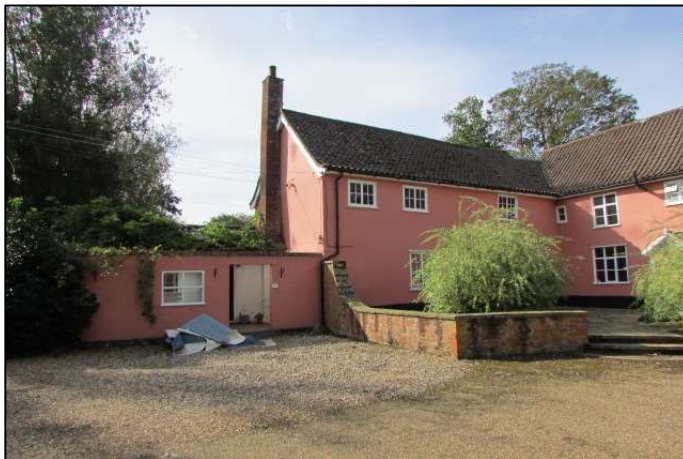
Figure 8 - Later extension & enclosed yard adjoining no. 1.
