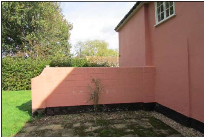
Figure 11 - Oil tank enclosure looking toward the barn.
