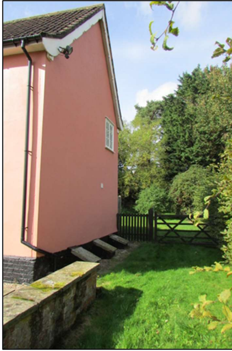
Figure 7 - North gable of no. 2.
