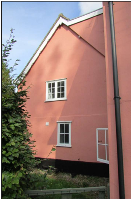
Figure 14 - South gable of no. 2.
