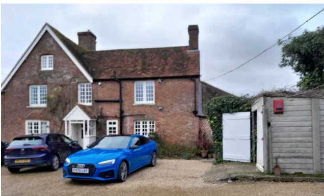
Inhurst Farmhouse - East elevation
