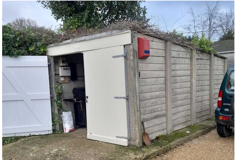
Concrete garage to be demolished
