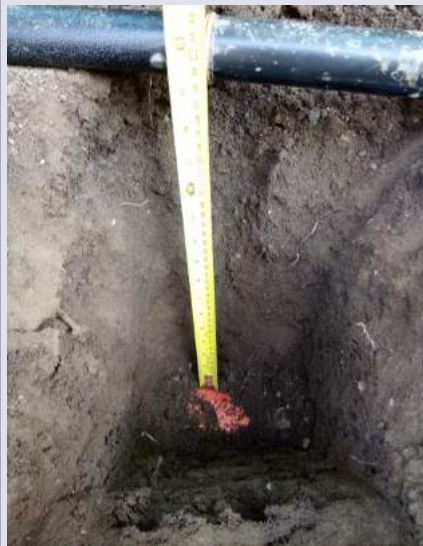
V114 geotextile in place, cover soil thickness 0.40m
