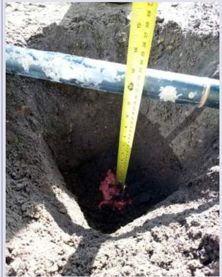
V103 geotextile in place, cover soil thickness 0.30m
