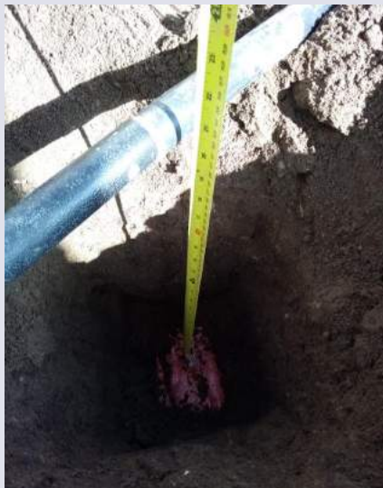
V105 geotextile in place, cover soil thickness 0.57m
