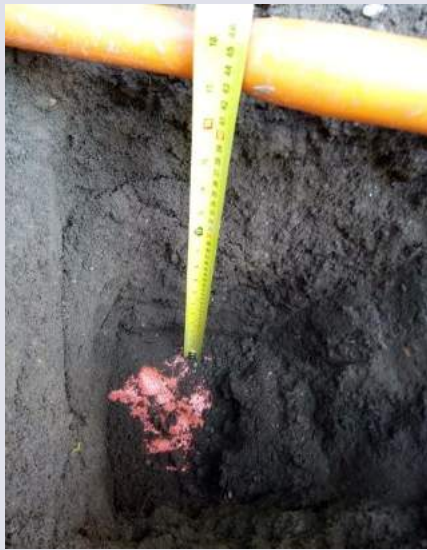
V110 geotextile in place, cover soil thickness 0.45m
