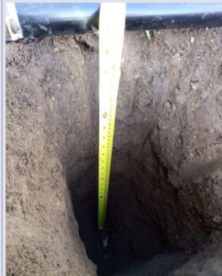
V106 geotextile in place, cover soil thickness 0.72m
