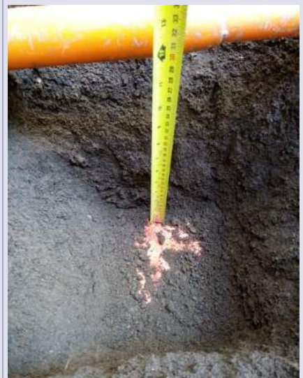
V109 geotextile in place, cover soil thickness 0.32m
