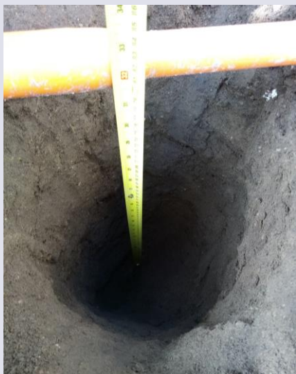
V107 geotextile in place, cover soil thickness 0.82m
