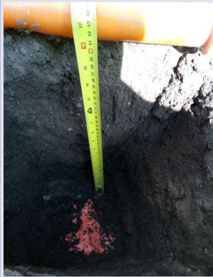
V111 geotextile in place, cover soil thickness 0.43m
