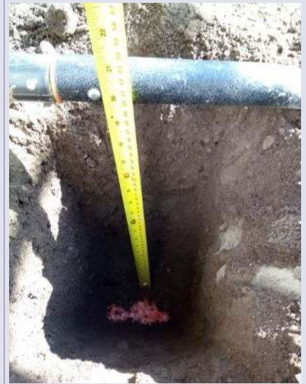
V112 geotextile in place, cover soil thickness 0.50m
