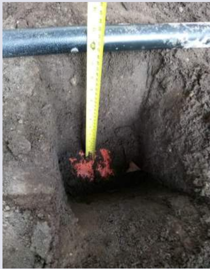
V102 geotextile in place, cover soil thickness 0.30m
