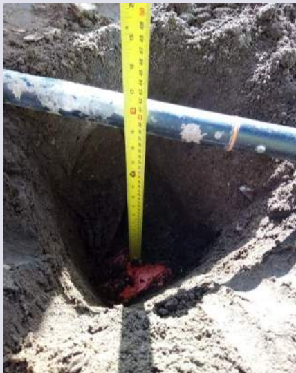
V104 geotextile in place, cover soil thickness 0.40m
