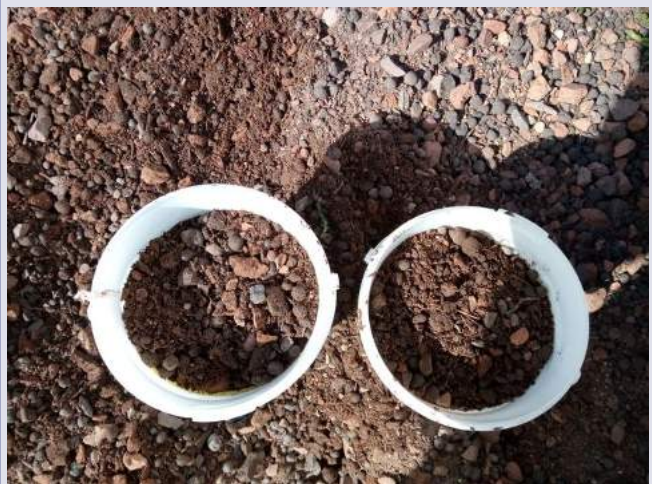
Imported topsoil – rooftop terrace garden
