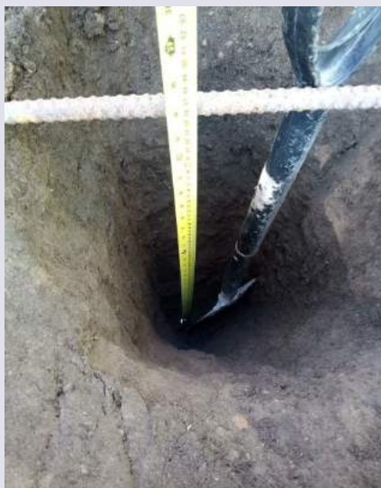
V108 geotextile in place, cover soil thickness 0.86m
