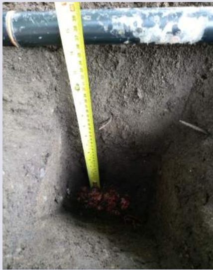
V101 geotextile in place, cover soil thickness 0.37m
