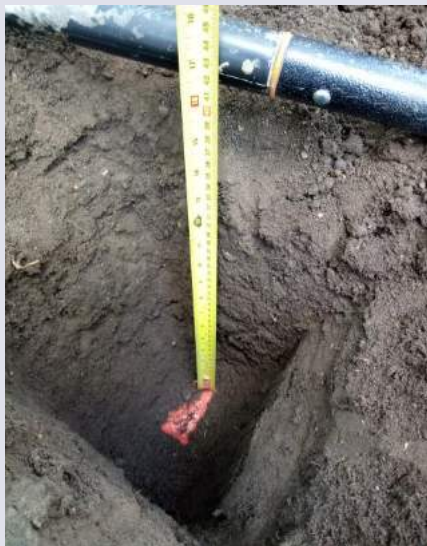
V113 geotextile in place, cover soil thickness 0.43m
