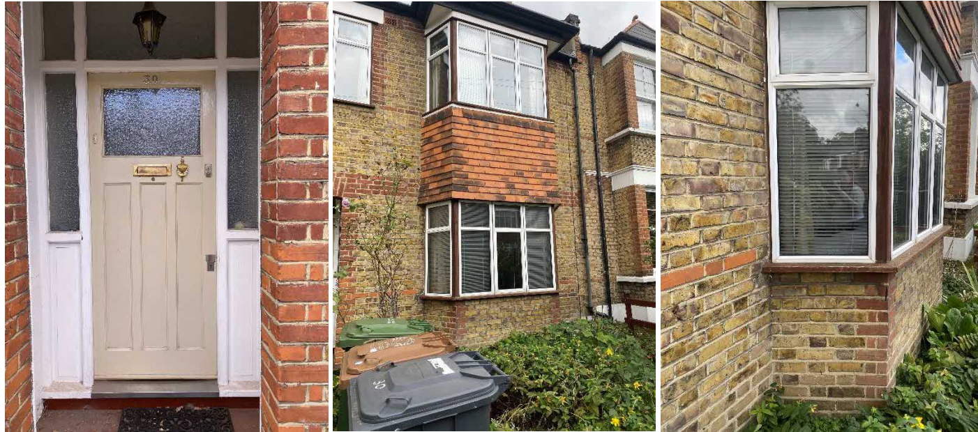
Existing front door and windows at 30 Manor Lane
