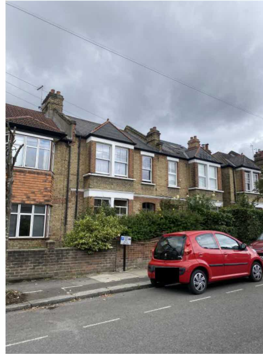
26 and 28 Manor Lane – original dwellings
