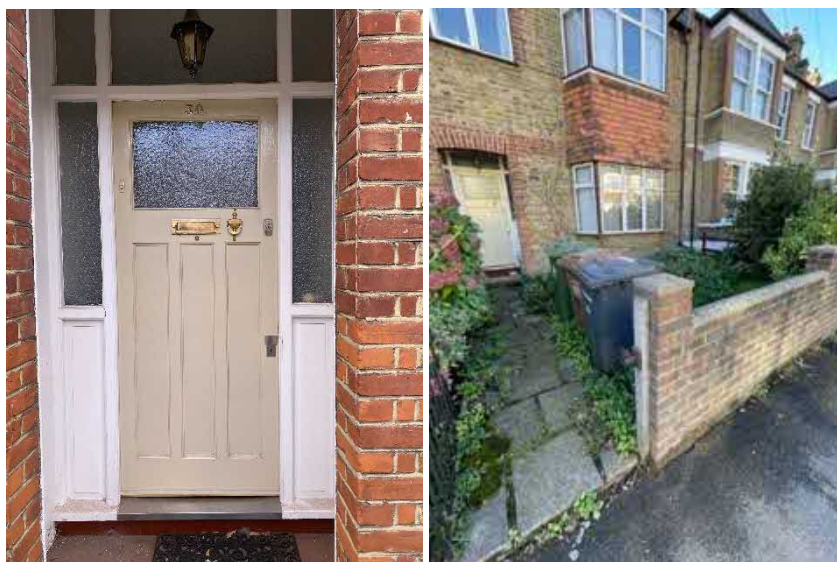
Existing front of 30 Manor Lane showing boundary wall, path, garden area and refuse and recycling bins, door and surround and windows.
