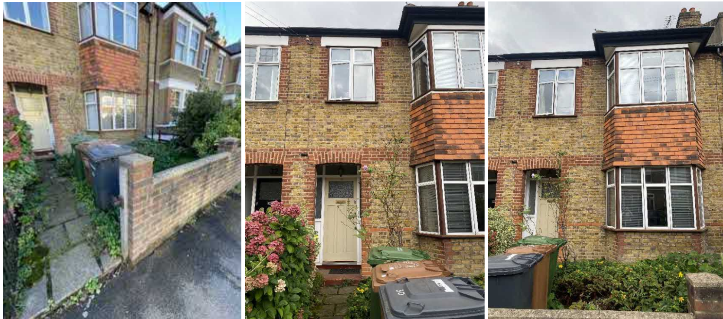
Existing front elevation of 30 Manor Lane
