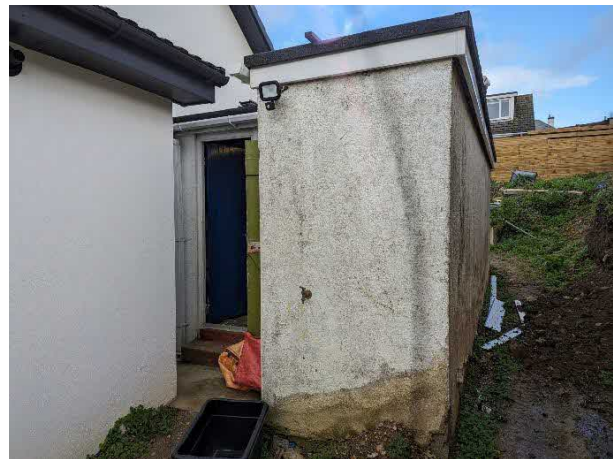
Photo 2. Showing the garage from the rear
