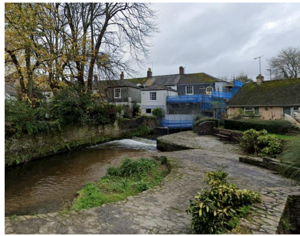
Figure 5. Rear elevation from Wilkes Walk to the southeast of the site
