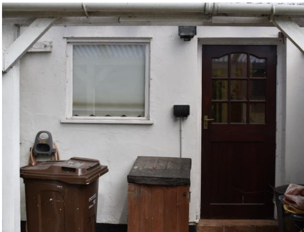
Figure 4. Lean-to extension/store at rear of building
