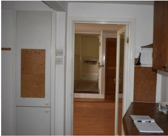
Figure 6. Partition wall between kitchen and dining room
