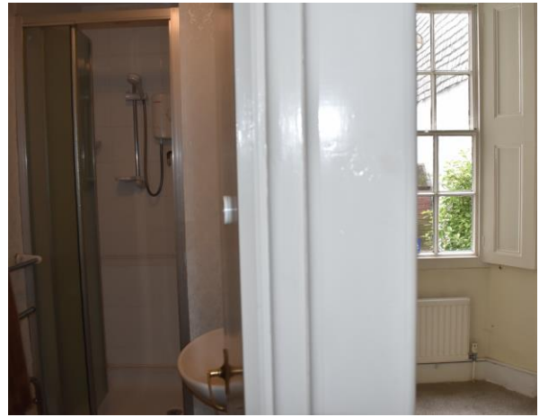
Figure 9. Modern shower room subdividing reception room on ground floor
