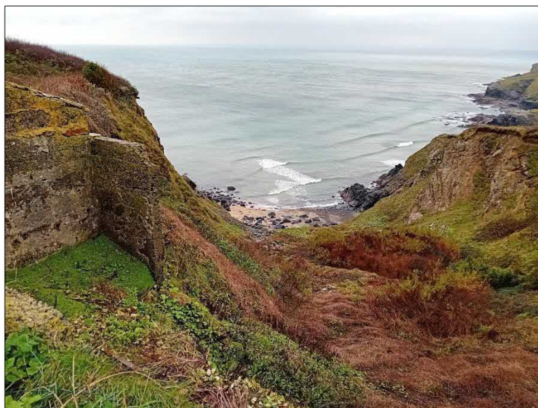
Figure 05: Sandy Pedn-y-ke – the ‘collapse lobe’ adjacent to the access track, derelict structure in foreground. Image taken from the unnamed access track, looking west.
