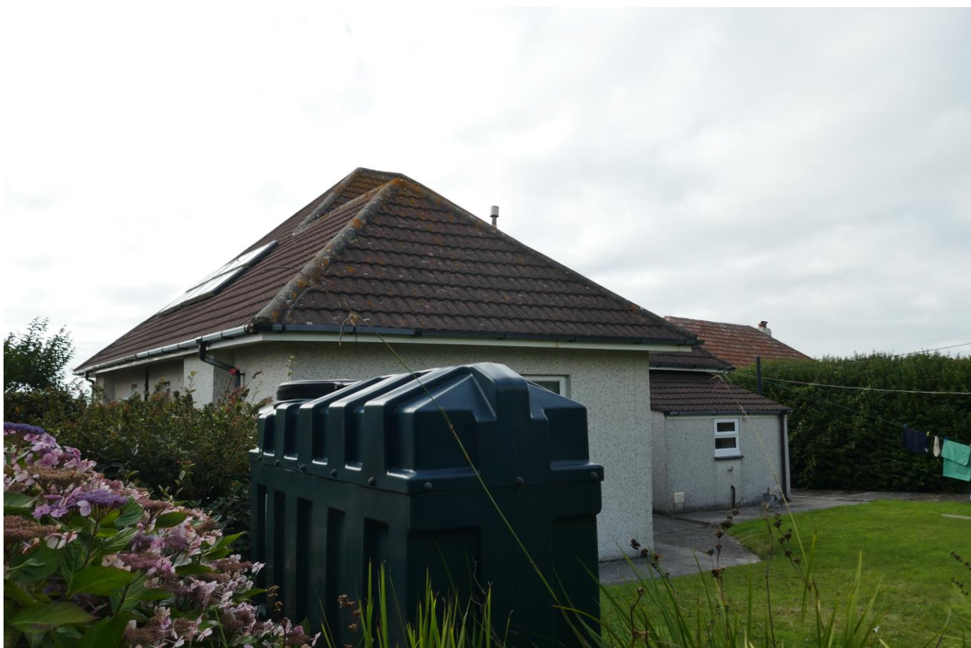
Figure 3. Southern and eastern aspects of the building.
