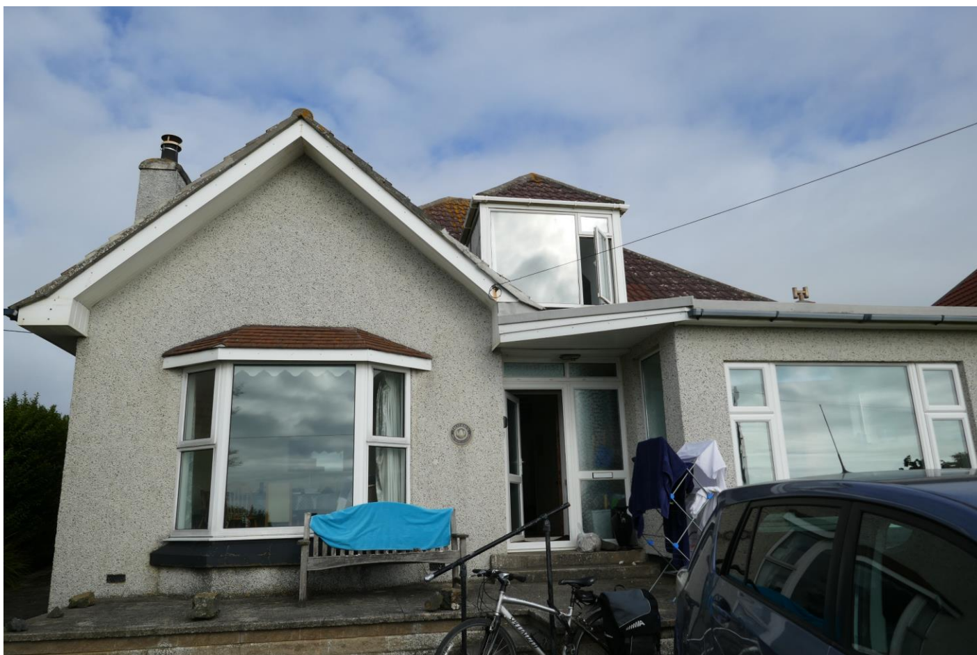
Figure 1. Western aspect of the building.
