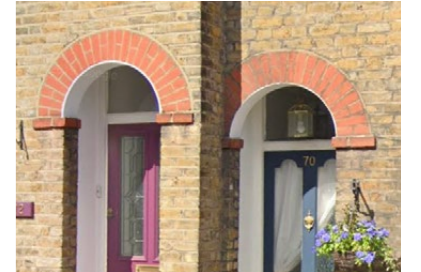
(A) Recessed entrance and arched entrances
