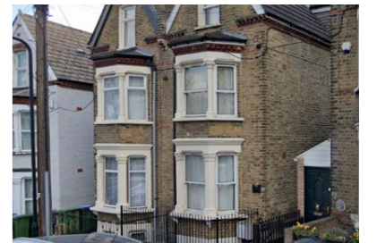
(C) Painted timber windows
