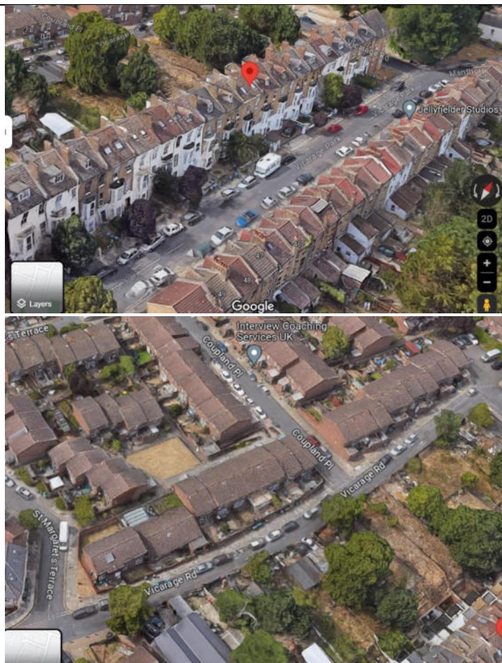
To show the consistent roof design of the adjacent roads
