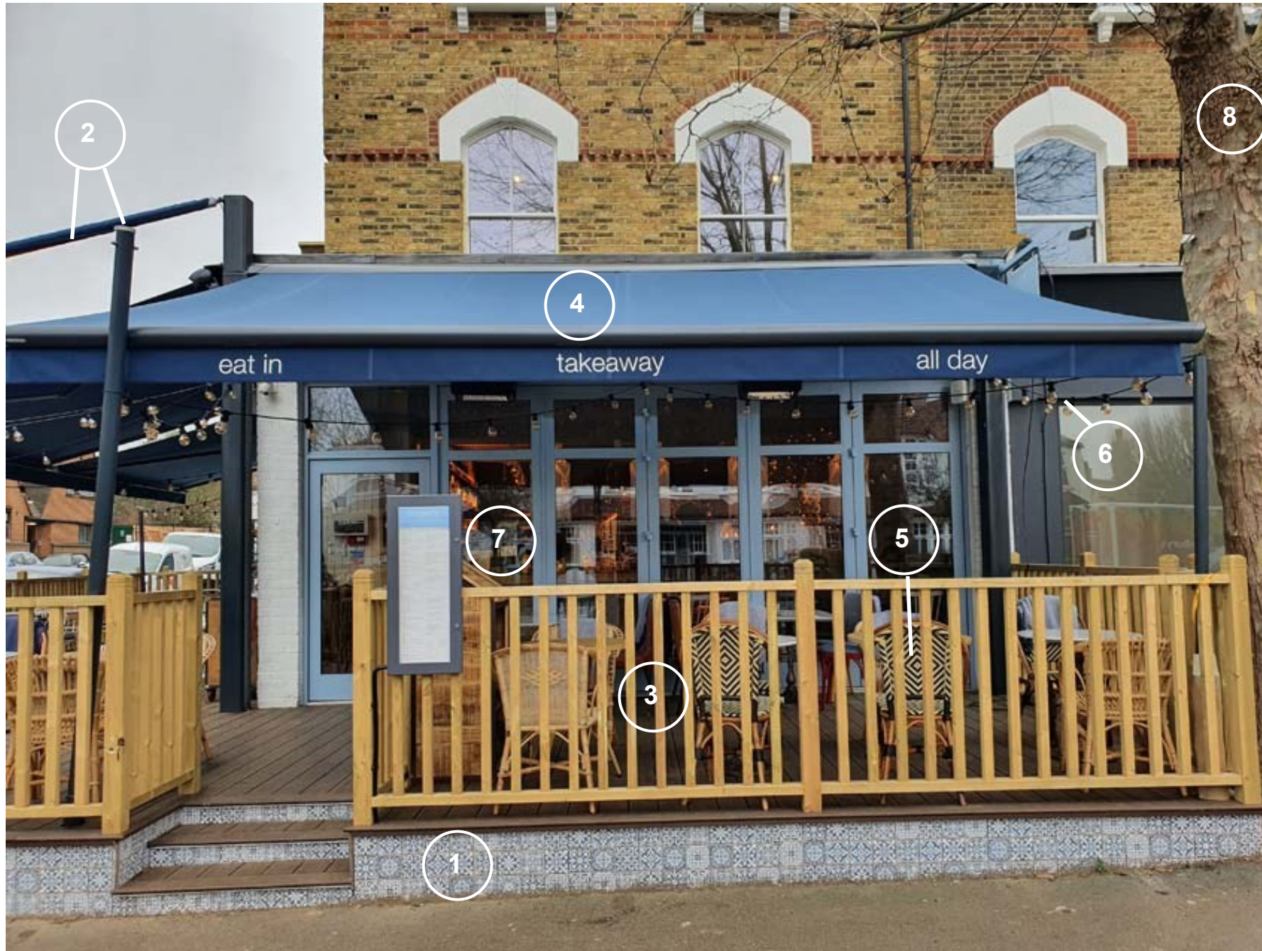
Image 03. Current Megan's unit. The annotation which is listed item 2.02 show the elements that are adapted, removed and retained.
