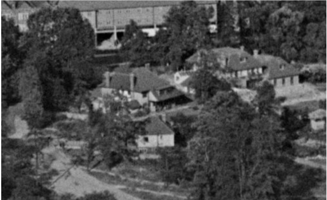
Figure 5: Aerial view captured in June 1931, taken from the southwest. Source: Britain from Above website [EPW035556] Housing at Arnos Grove, Christ Church and environs, New Southgate.
