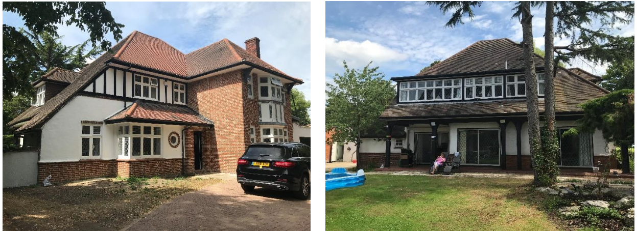
Figure 2: No. 21 the Green – front elevation (left) and elevation to rear garden (right)
