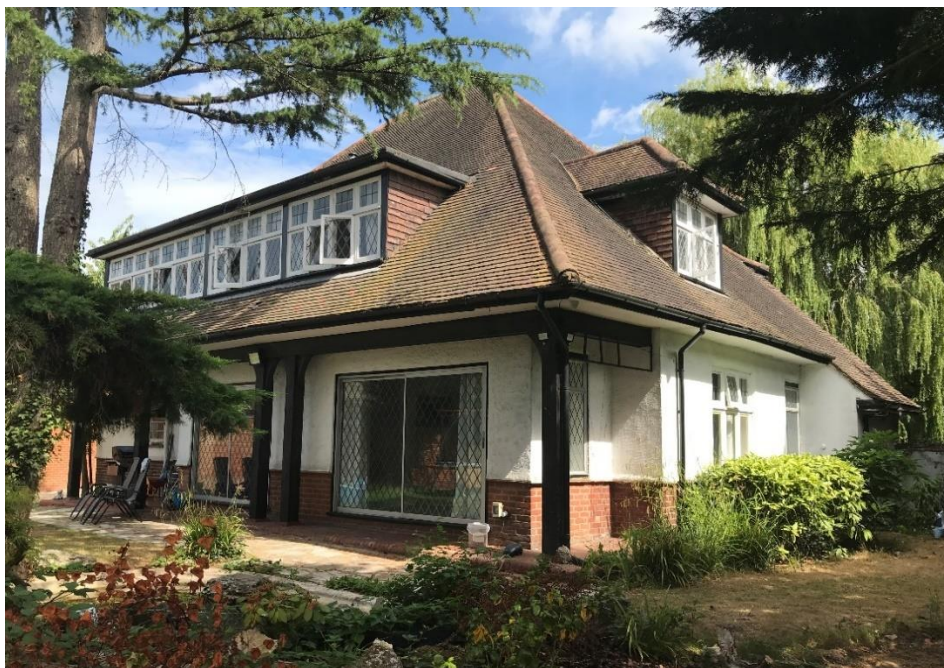
Figure 8: View of the rear elevation from the south
