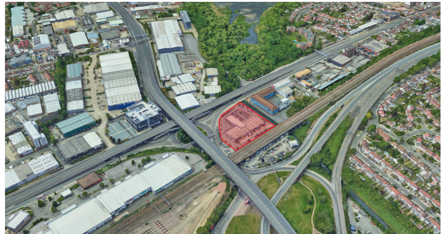
Aerial view looking west - Google images
