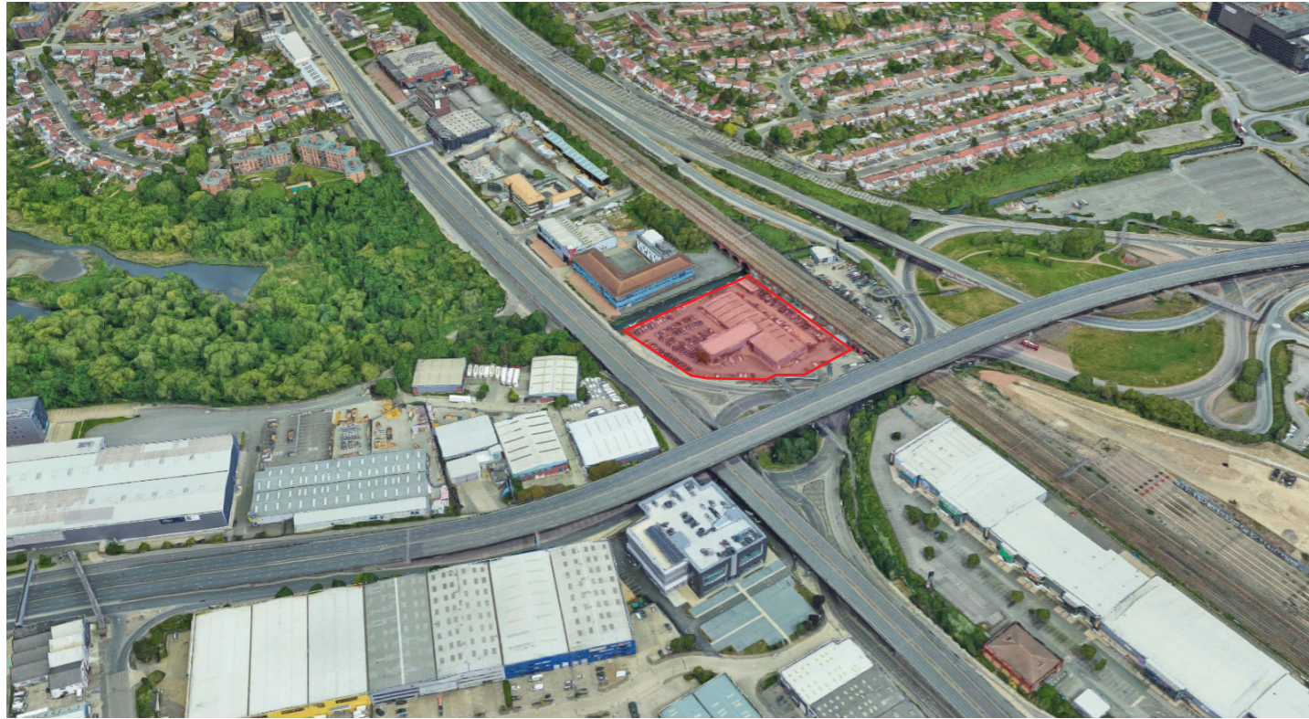
Aerial view looking north - Google images
