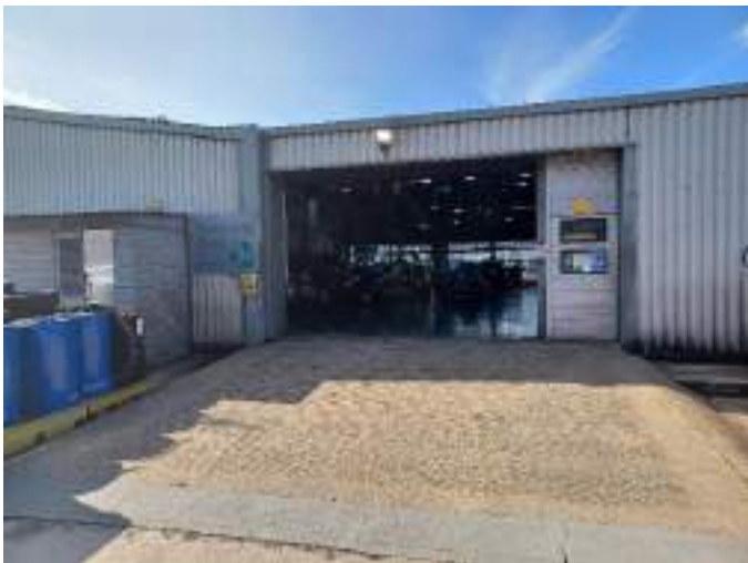
Photo 7: Service garage at the rear of the dealership in the north of the site
