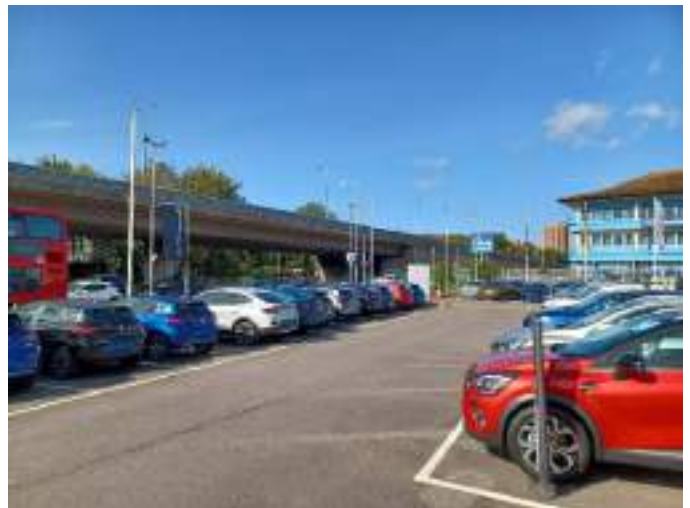
Photo 12: Viewing the A5 flyover to the west of the site
