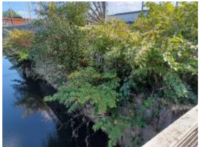
Photo 16: Visible Japanese Knotweed on the north western site boundary
