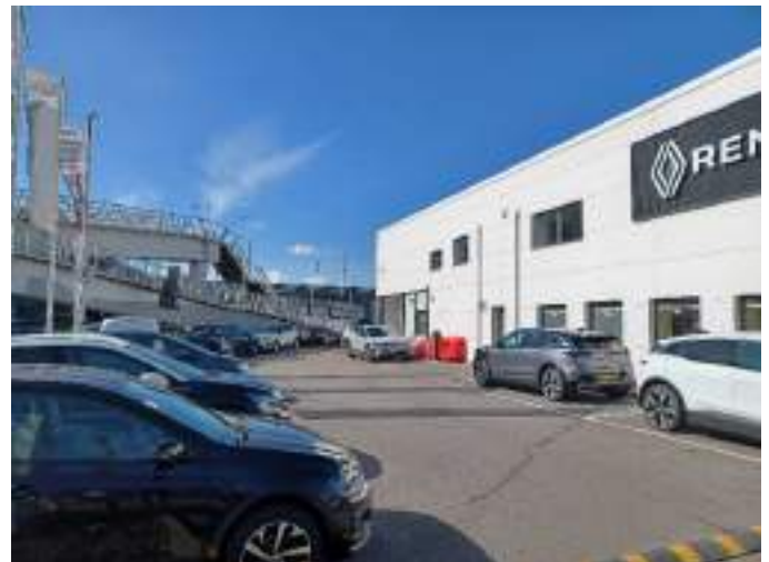
Photo 4: Parking to the south east of the dealership.
