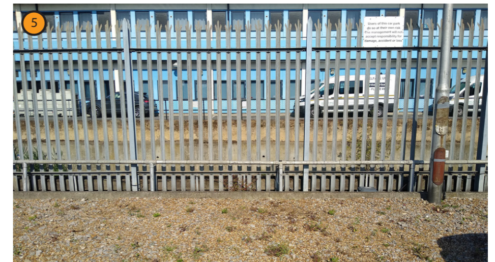
Northwest boundary: metal palisade fencing and lack of soft landscaping
