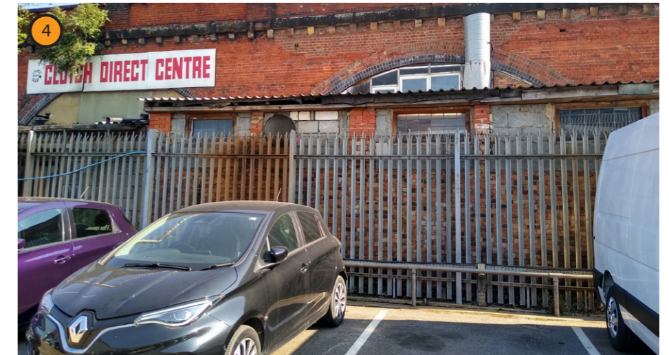
Northeast boundary: metal palisade fencing
