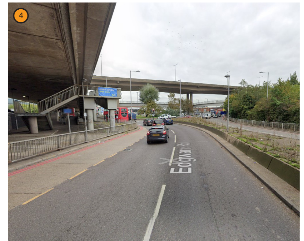
Northbound approach along Edgware Road - Google street view
