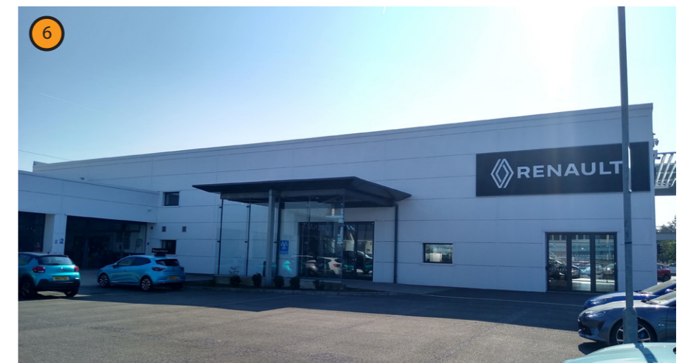
Existing north entrance into the building
