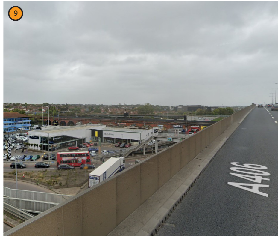
Eastbound along the raised section of the North Circular Road - Google street view
