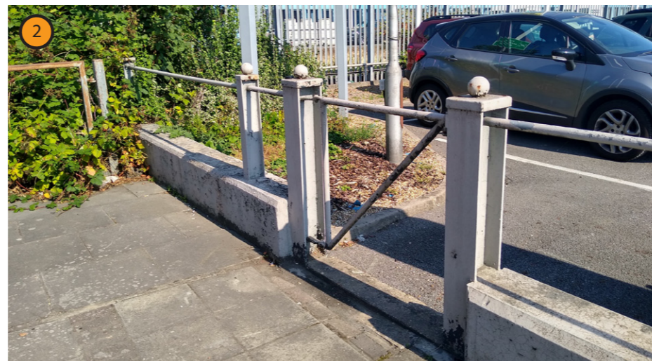
Southwest boundary treatment: low concrete wall with metal railing and posts
