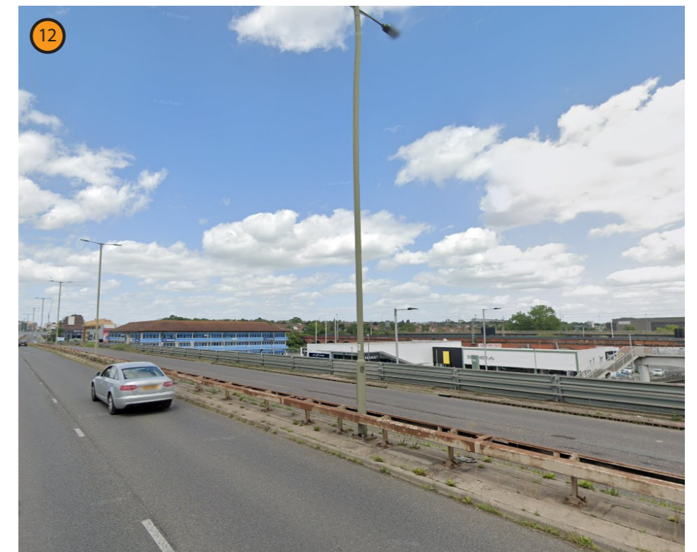
Northbound along the raised section of Edgware Road - Google street view
