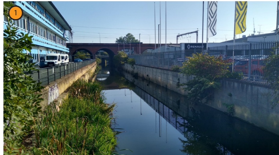
River Brent running along the northwest site boundary
