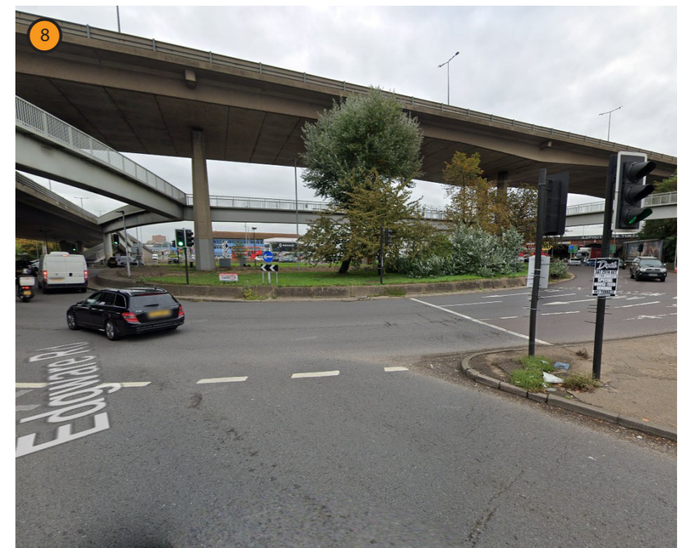
Northbound approach to Staples Corner west roundabout - Google street view
