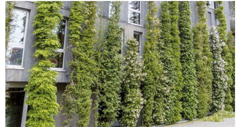
Green wall screening from ground level planting
