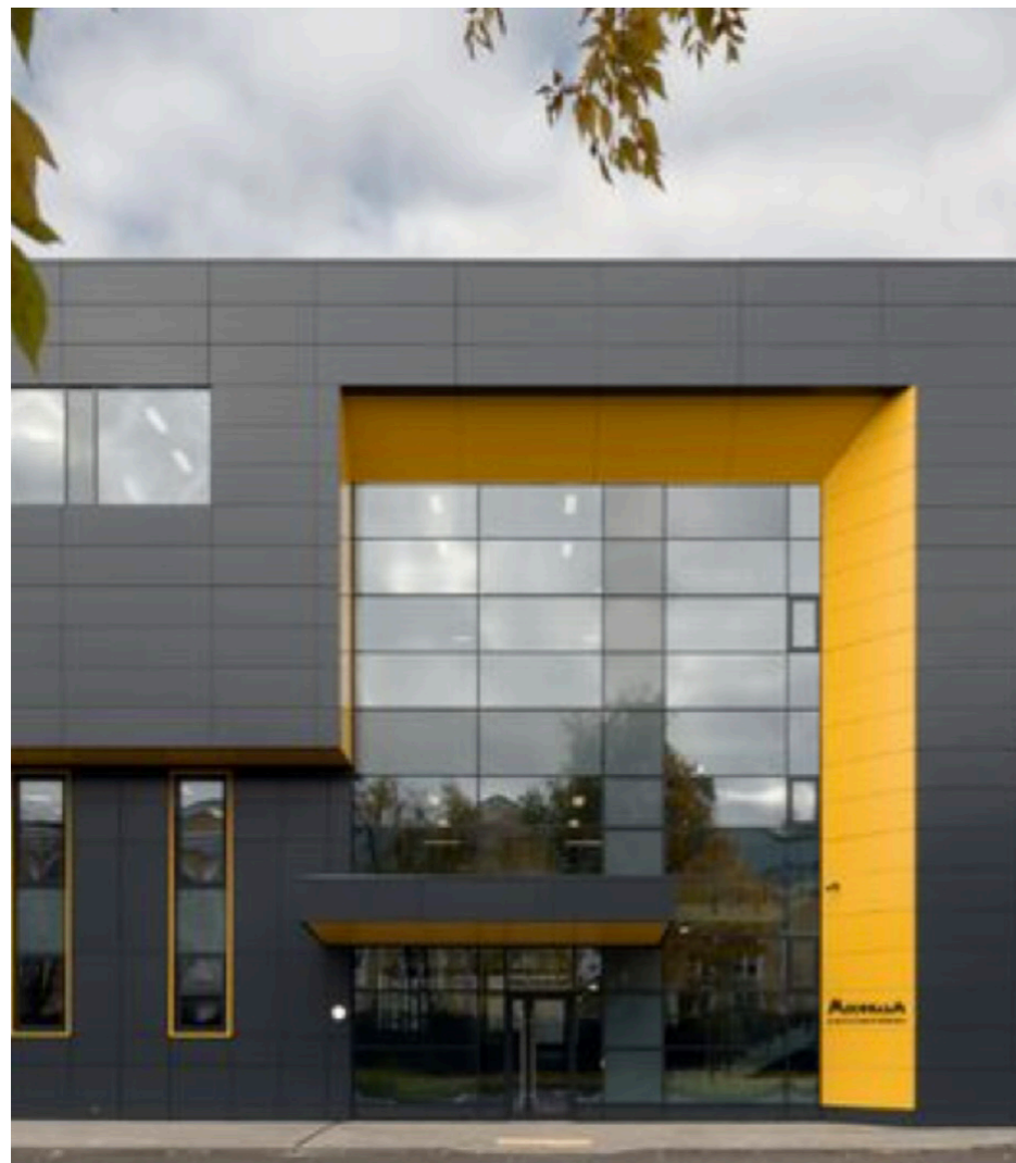
A deep cut out to form the main entrance into the building
