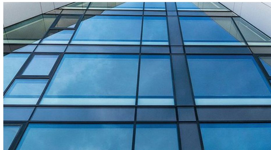
Dark grey curtain walling system with opaque glass spandrel panel
