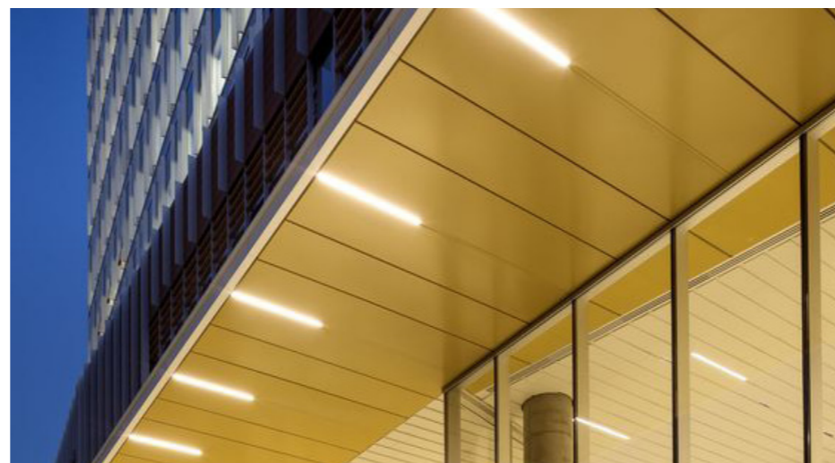
Yellow metal rainscreen cassette cladding system (lighting indicative only, to be developed)
