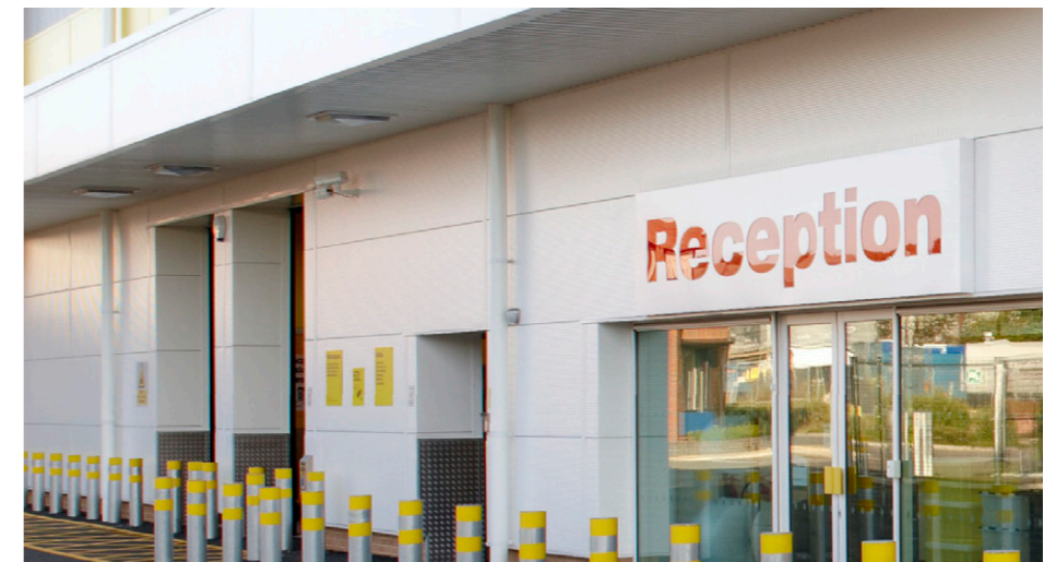
White composite insulated metal cladding to loading area
