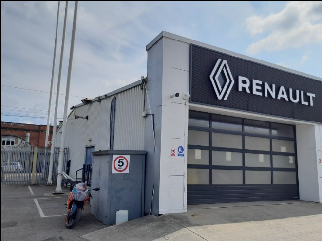
Photograph 1. Central building onsite.
