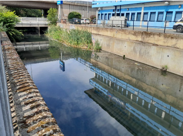
Photograph 2. Offsite River Brent, north of the red line boundary.
