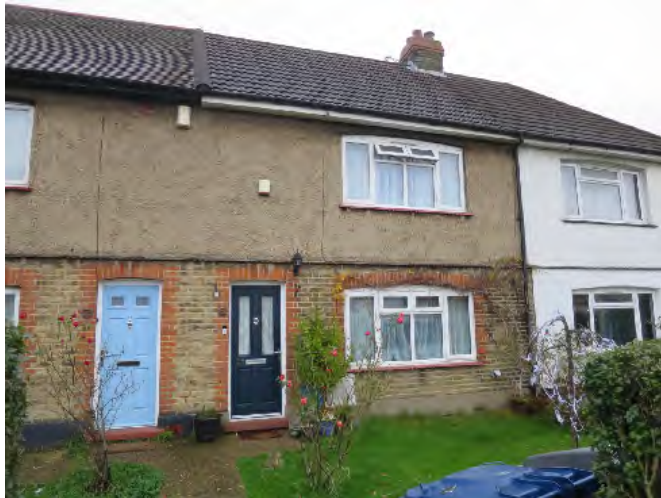
01 Existing property photo at 61 Clitterhouse Crescent, NW2 Front, as viewed from Clitterhouse Crescent, as at December 2023
