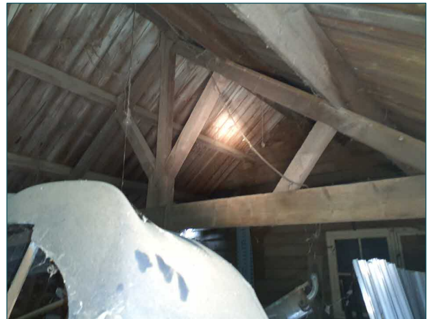
Photograph 4. Internal view of Building B1.
