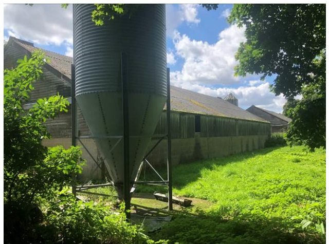
Photo 6: Building C – north eastern facades
