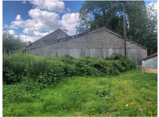
Photo 10: Building E – eastern façade, with bramble scrub growing alongside building
