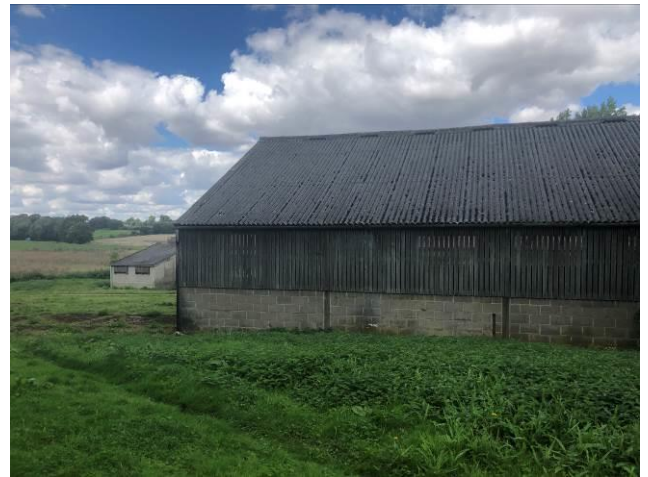
Photo 4: Building A – northern façade
