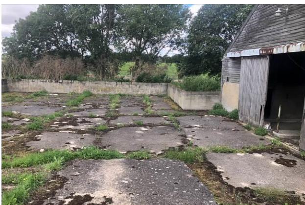
Figure 4: Existing concrete bunded area immediately west of Building C
