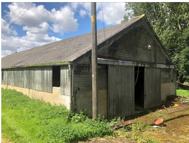
Photo 5: Building C – south eastern facades
