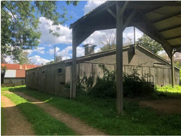
Photo 9: Building E – south western facades, with adjacent open sided barn
