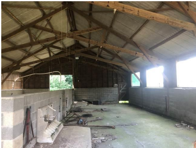
Photo 3: Building A – internal view
