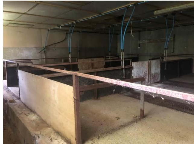
Photo 12: Building E – internal view
