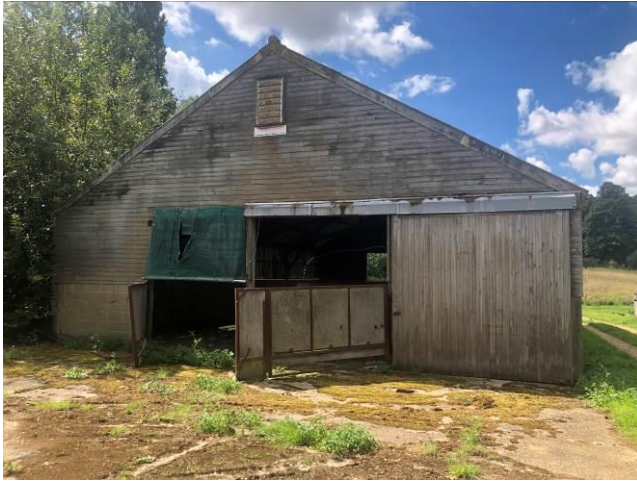
Photo 1: Building A - eastern gable end
