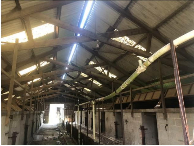
Photo 7: Building C – internal view
