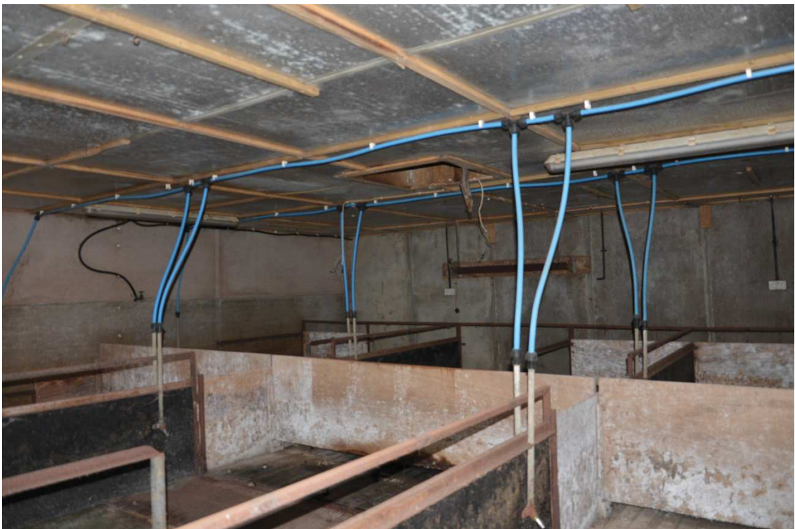
Photo 18 , internal view of building three, looking southeast.
