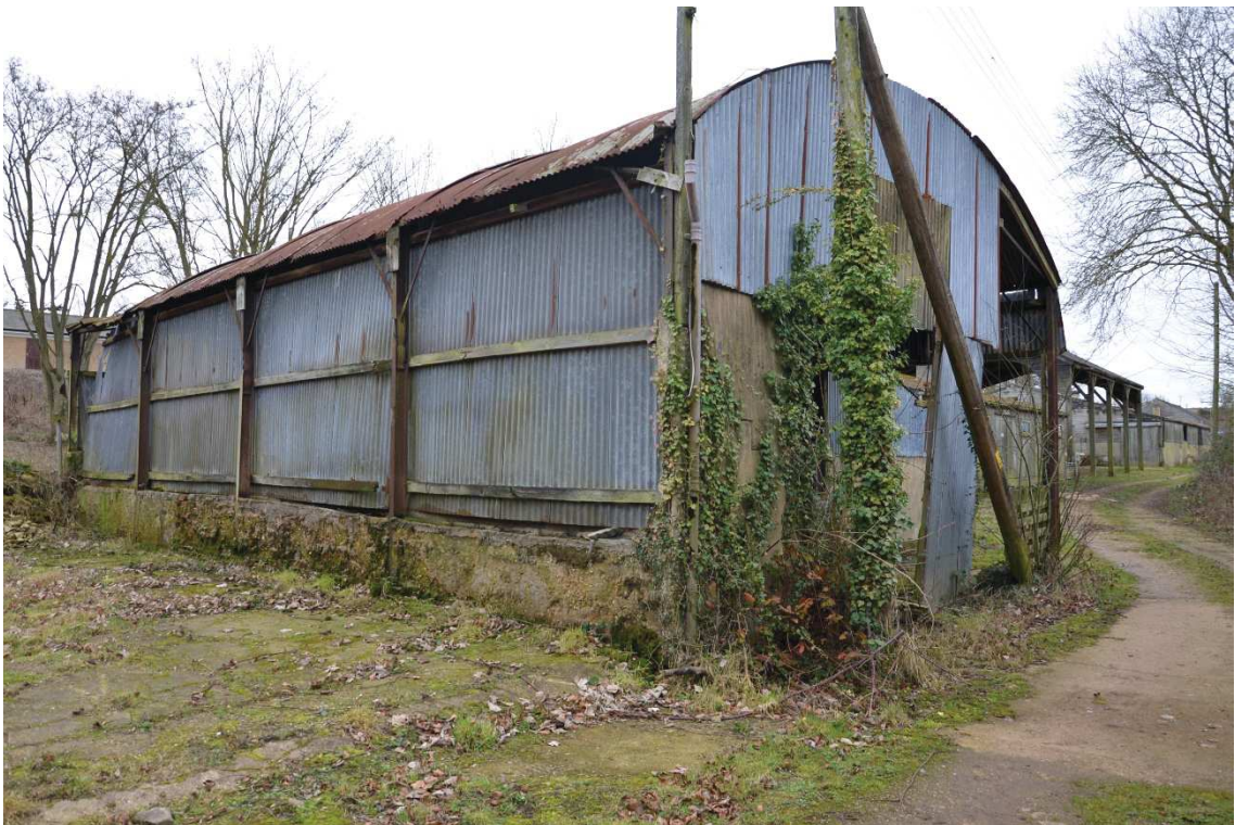
Photo 15 , external view of building two, looking southwest.
