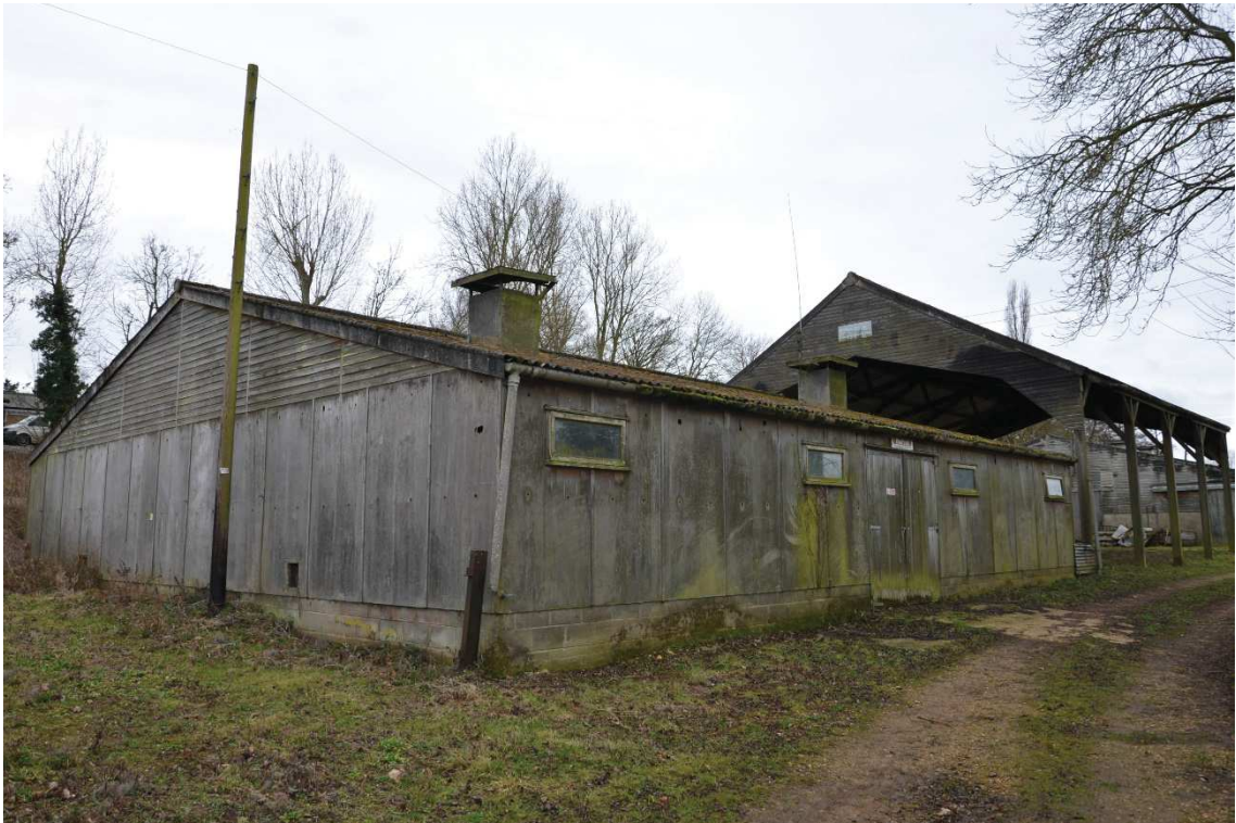
Photo 17 , external view of building three, looking southwest.
