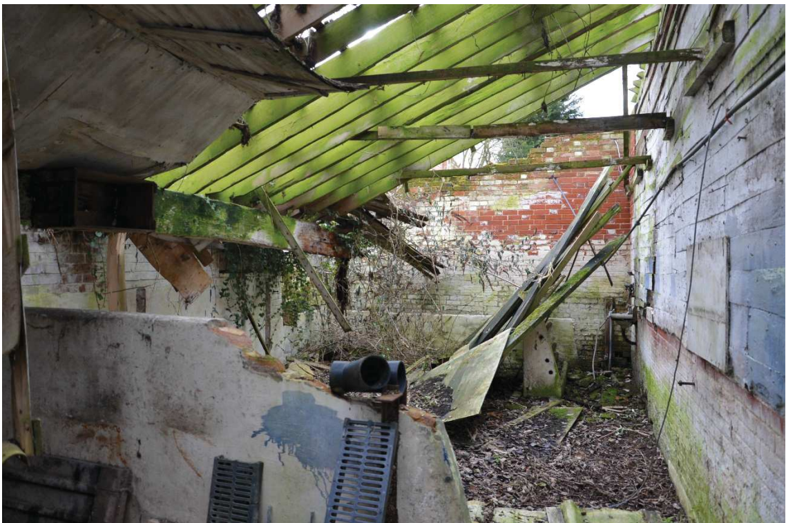
Photo 14 , internal view of building one, looking south.
