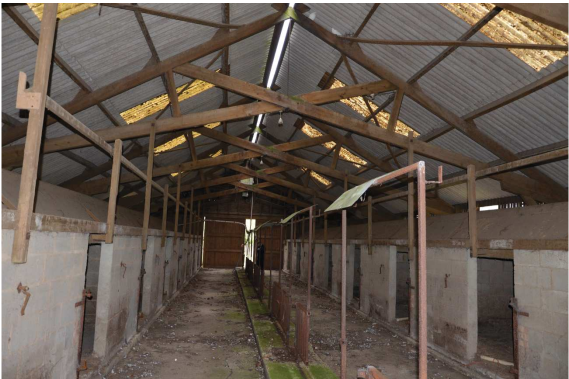
Photo 21 , internal view of building six, looking west.
