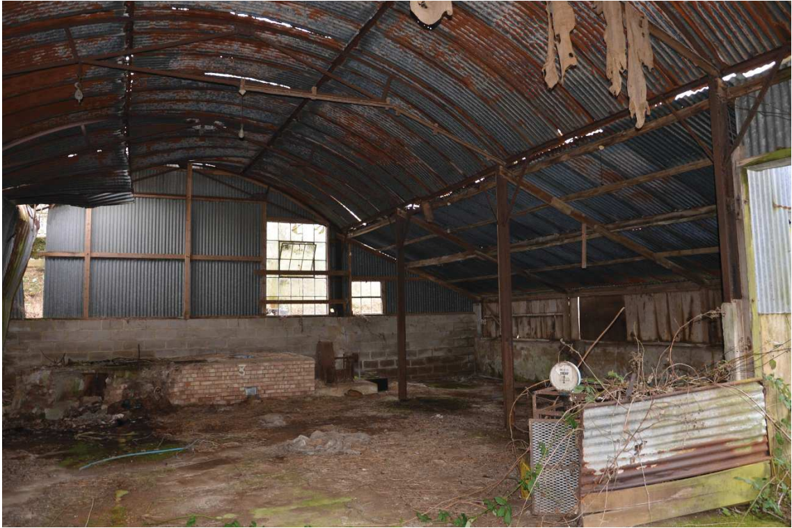
Photo 16 , internal view of building two, looking south.
