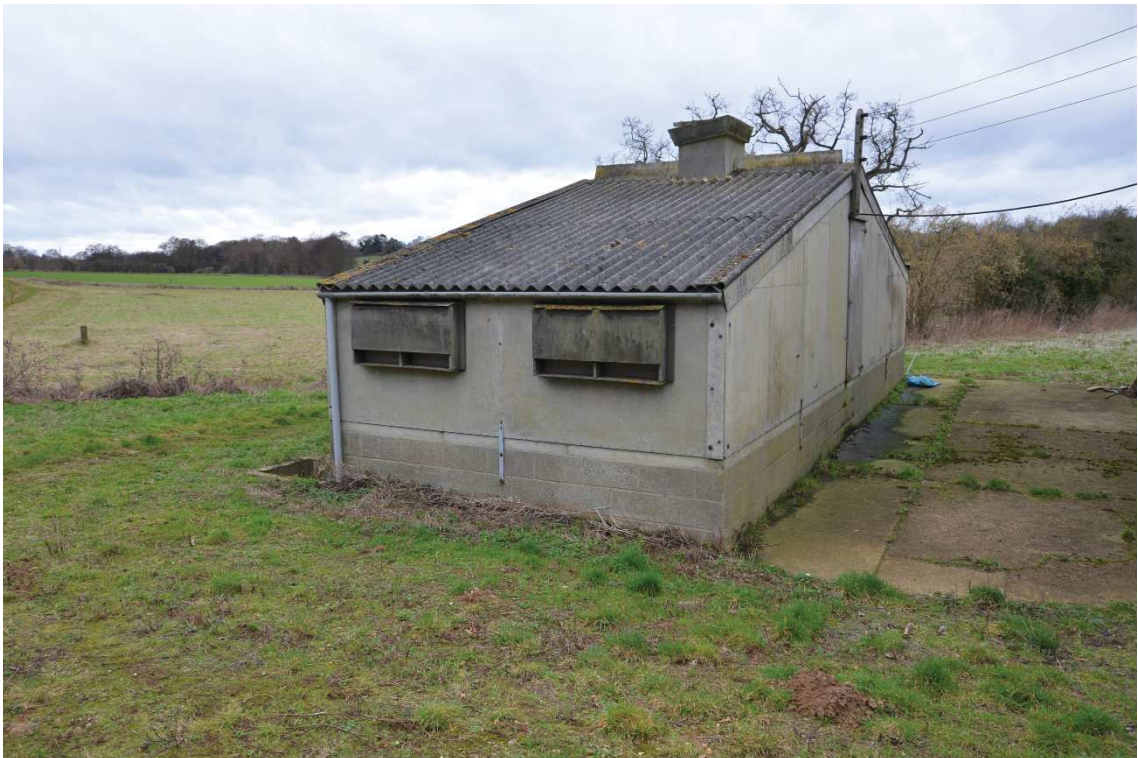
Photo 22 , external view of building nine, looking northwest.
