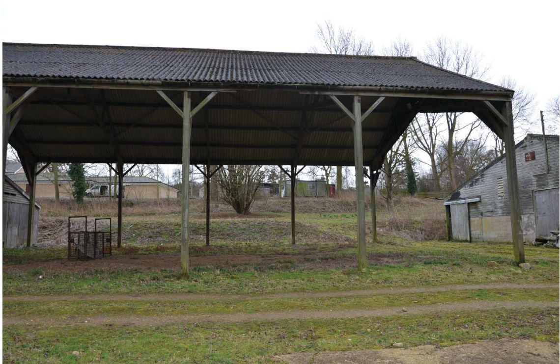
Photo 19 , view of building four, looking south.
