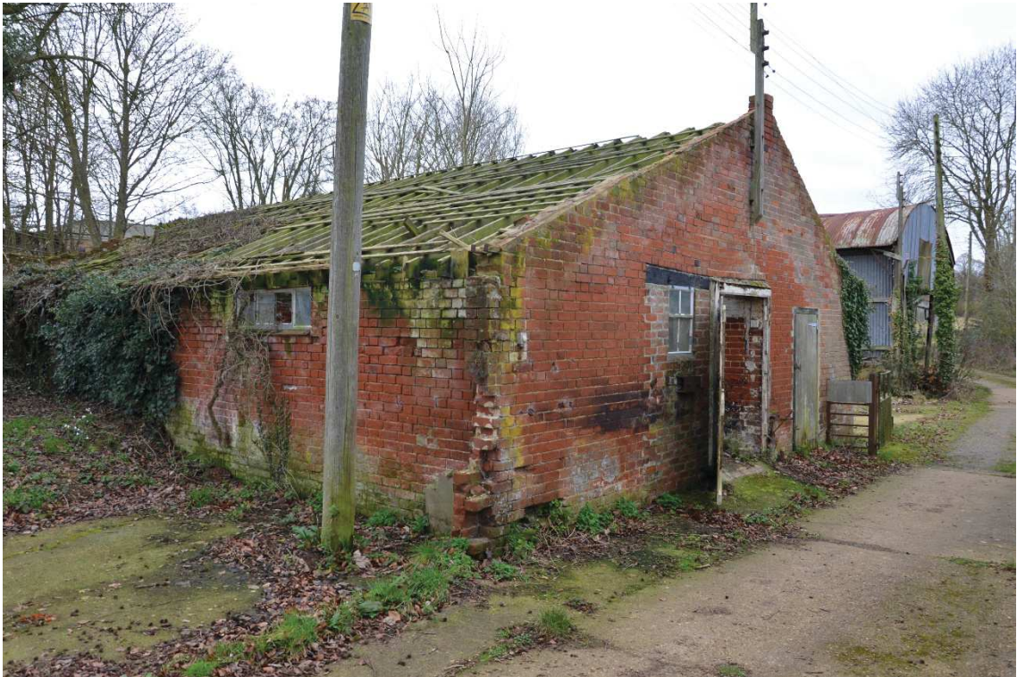
Photo 13 , external view of building one, looking southwest.
