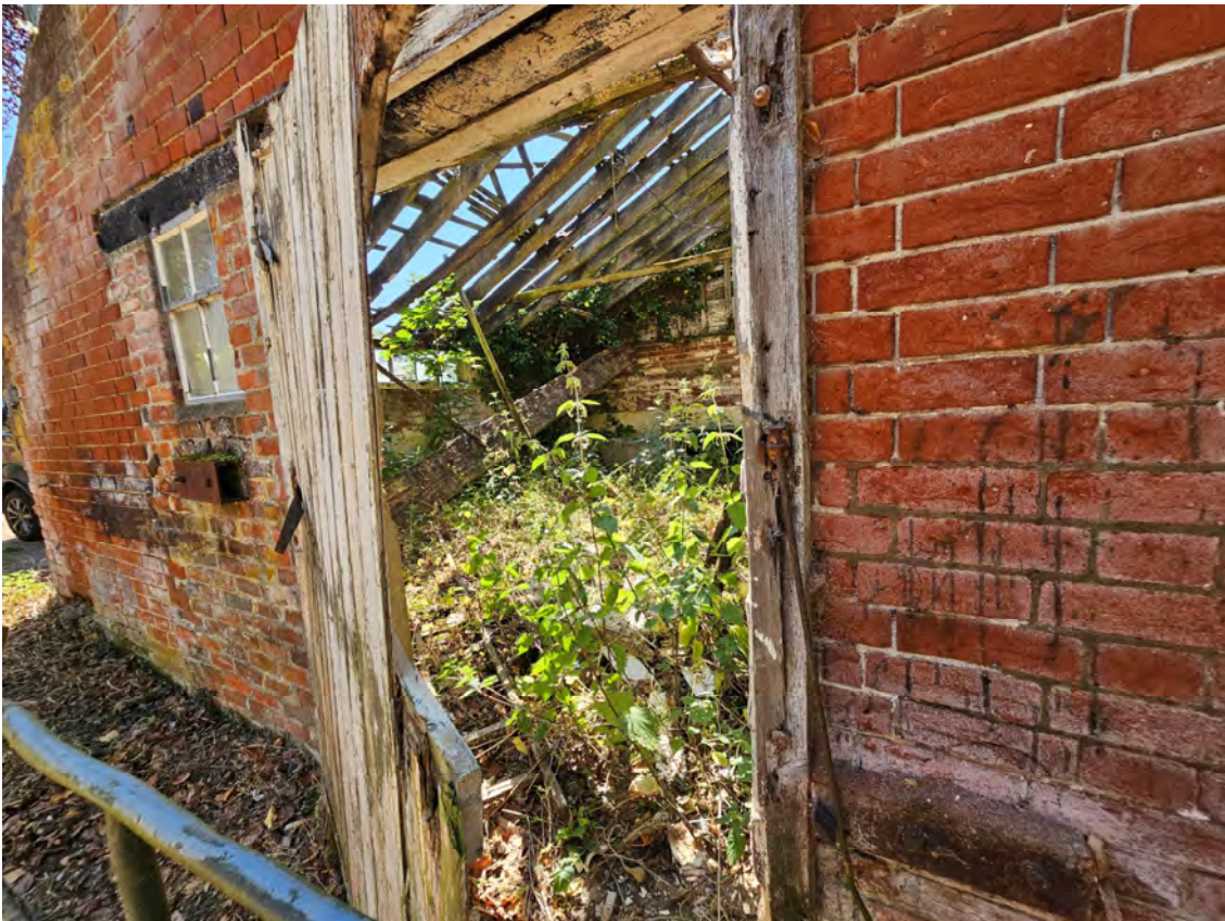
Photograph 3 : Inside the building.
