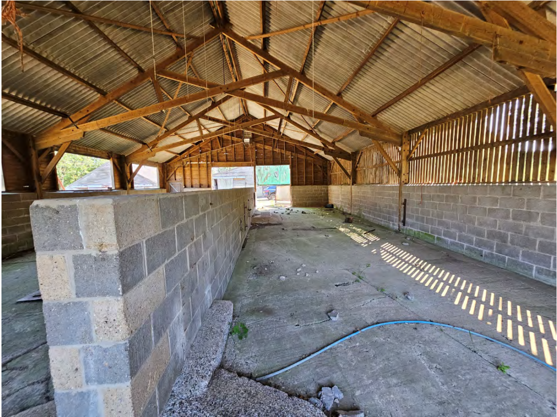
Photograph 14: View inside Barn A looking east.
