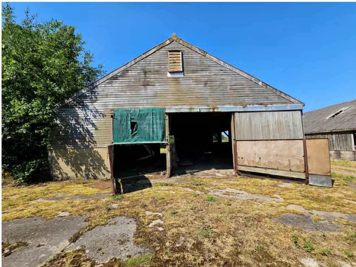
Photograph 13: East elevation of Barn A south of track.
