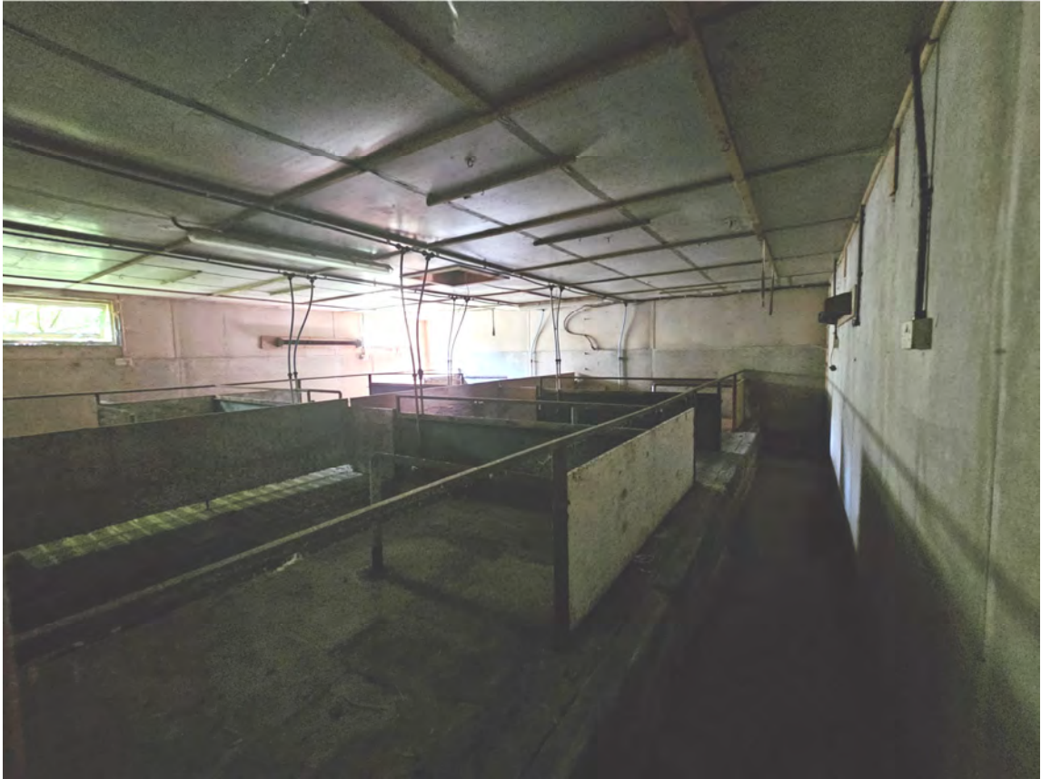
Photograph 8: View inside the rooms of the building.
