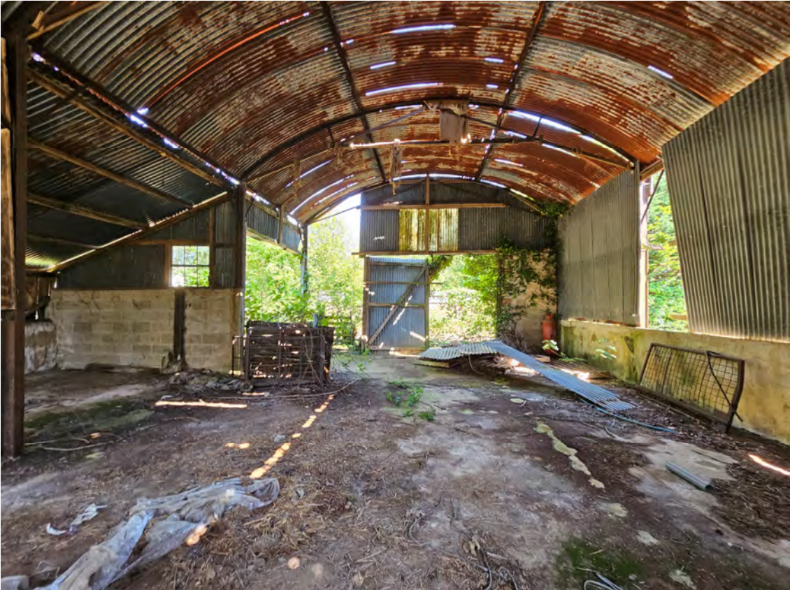
Photograph 5: View looking inside the Dutch barn.
