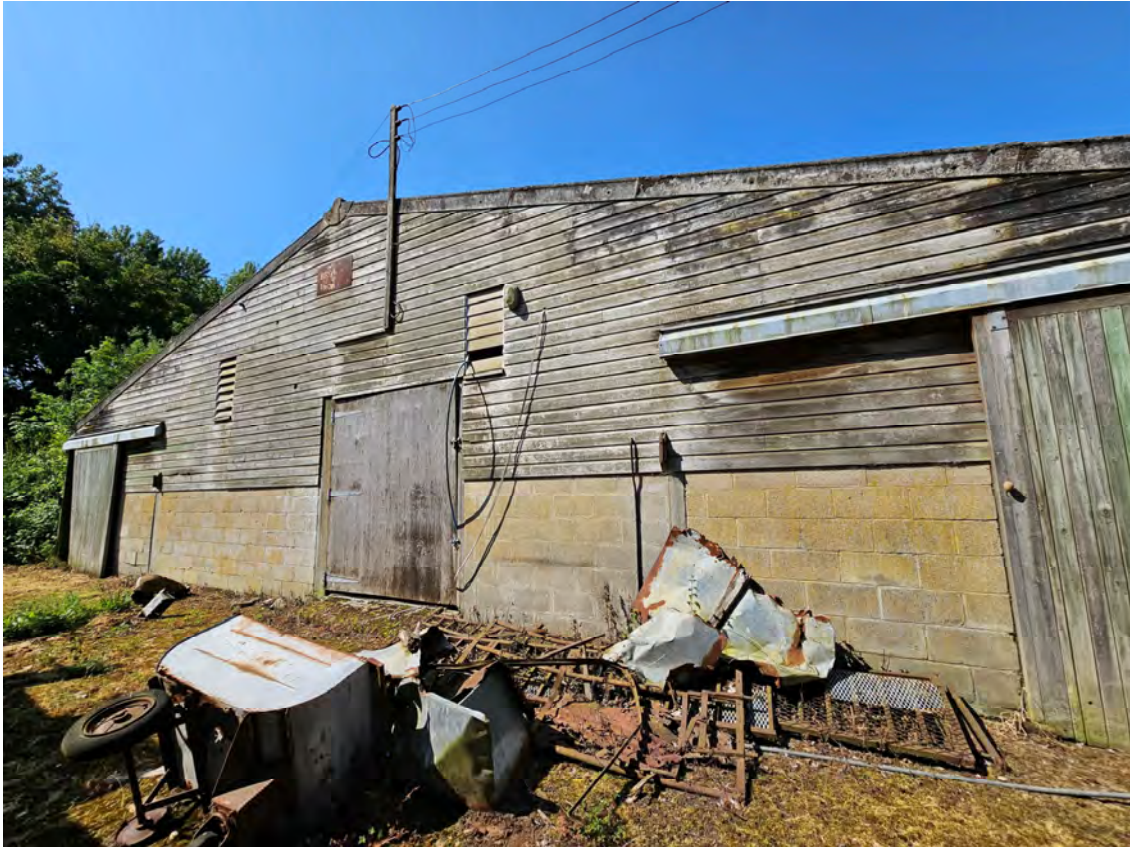
Photograph 10: Eastern end of Barn D south of track.
