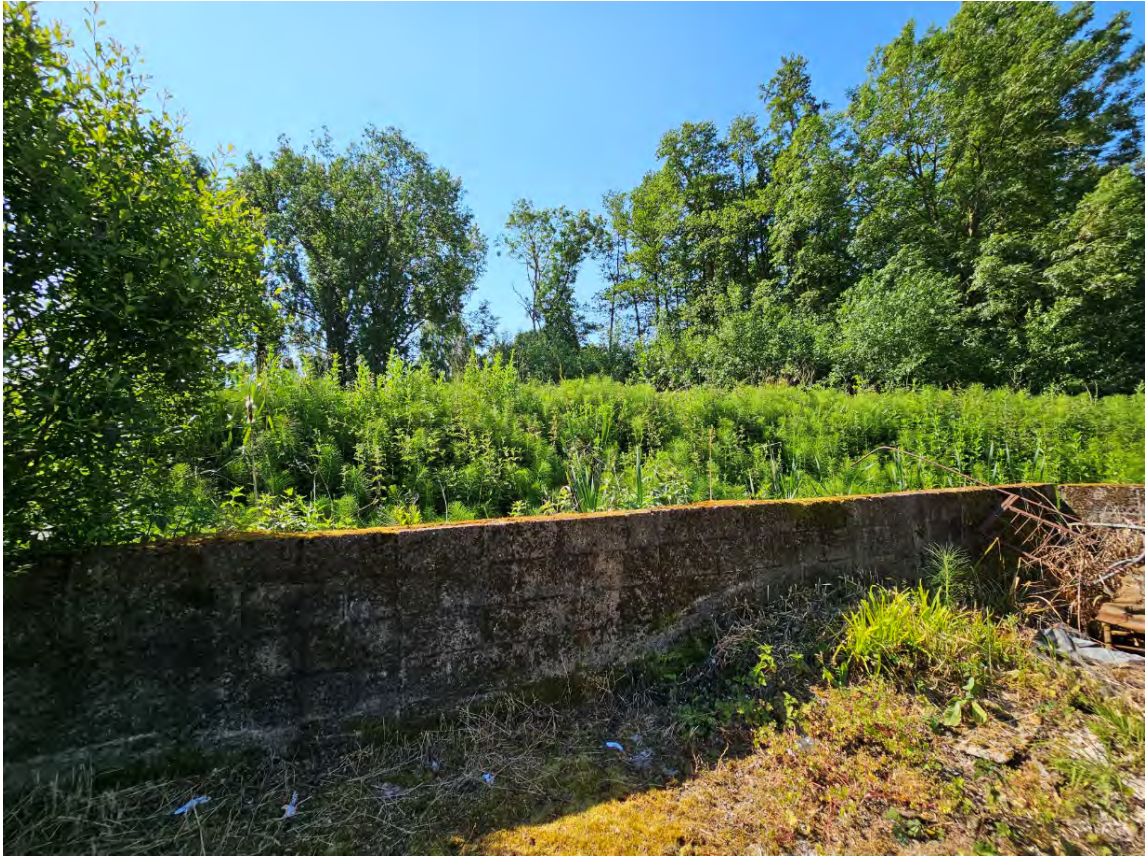
Photograph 12: View of the elevated land to the south of Barn D.
