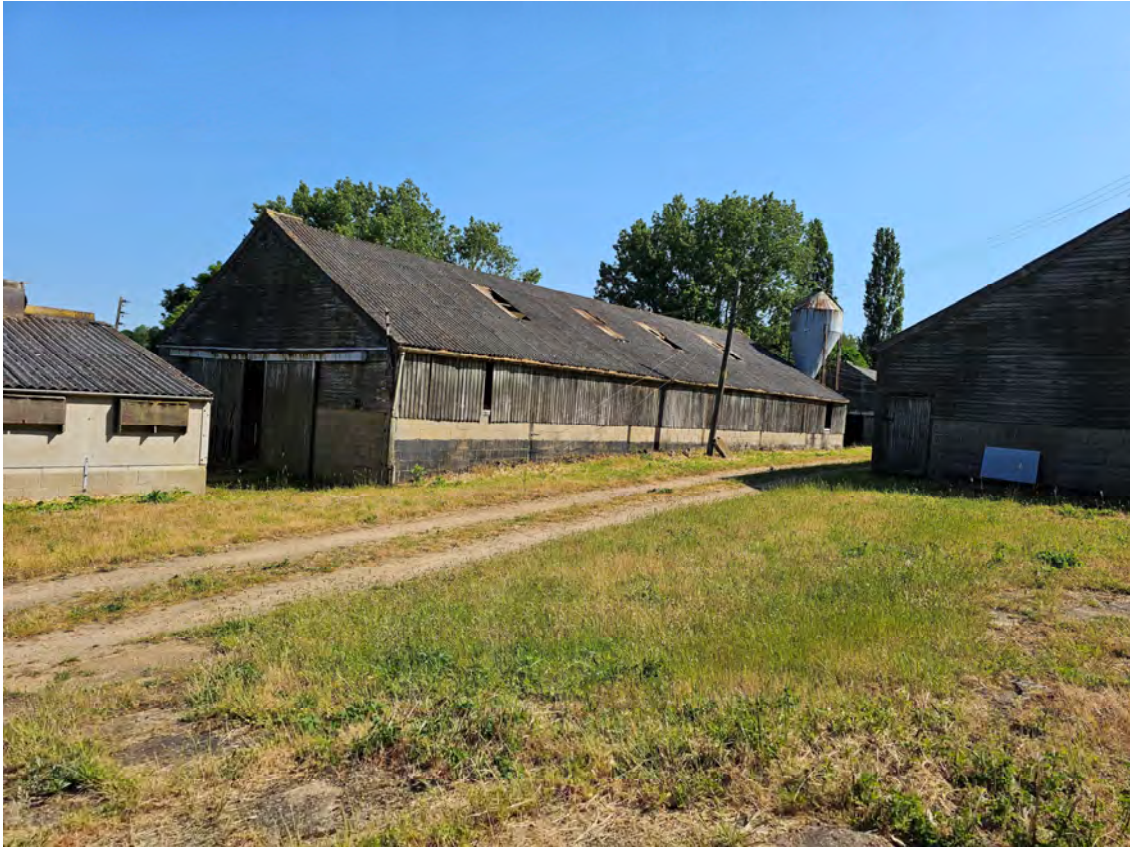
Photograph 18 : Barn B located on the north side of the track.
