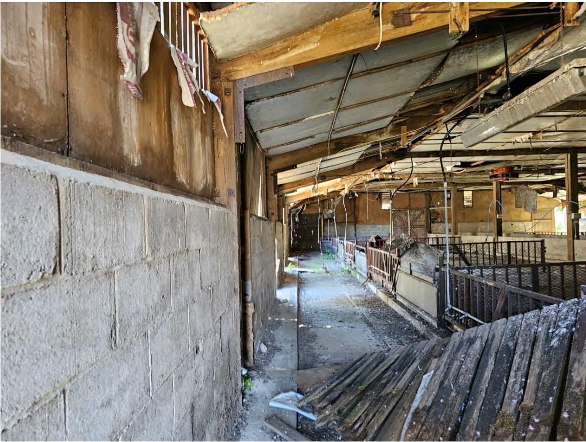
Photograph 11: View inside Barn D looking east.
