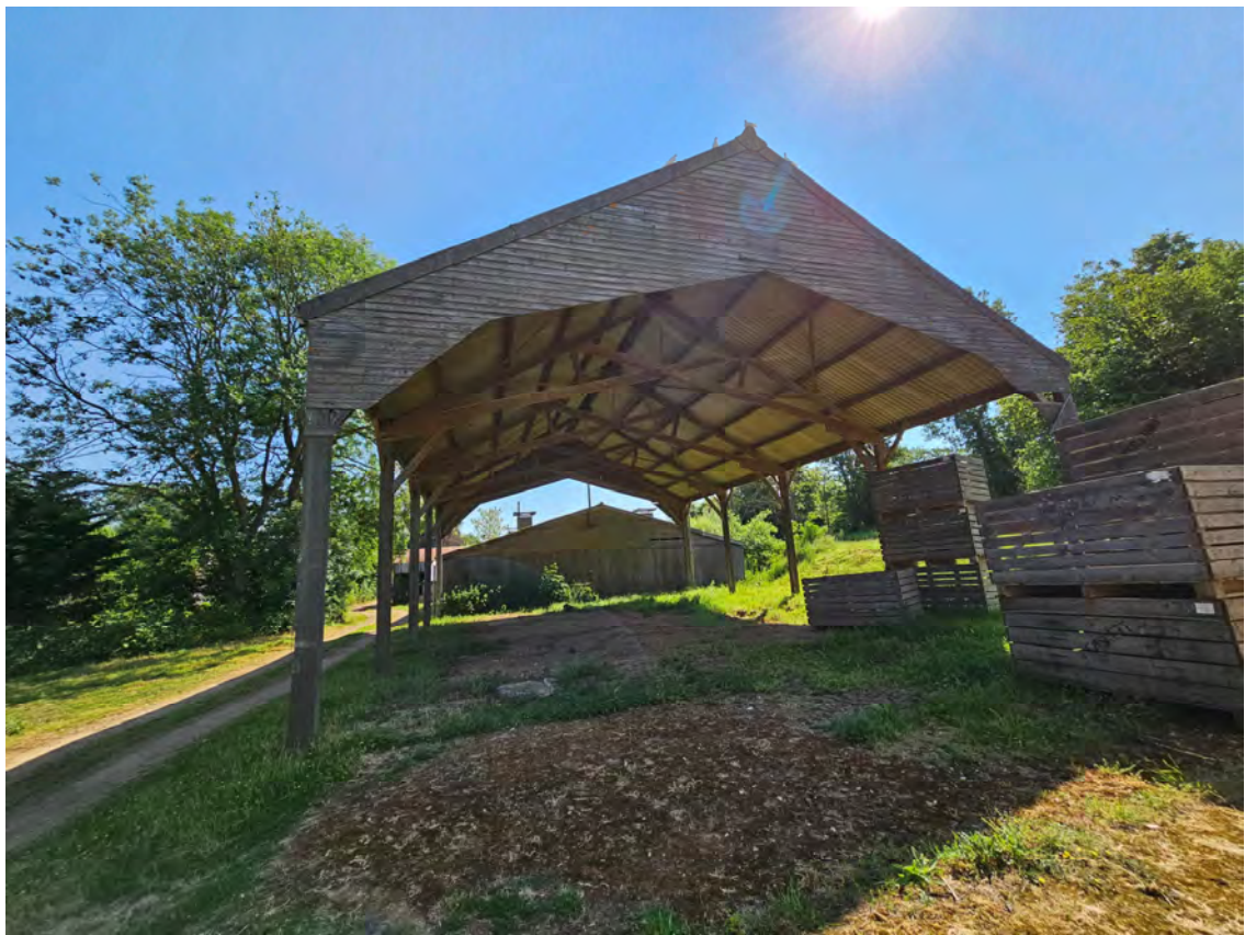
Photograph 9: Timber framed hay barn south of track.
