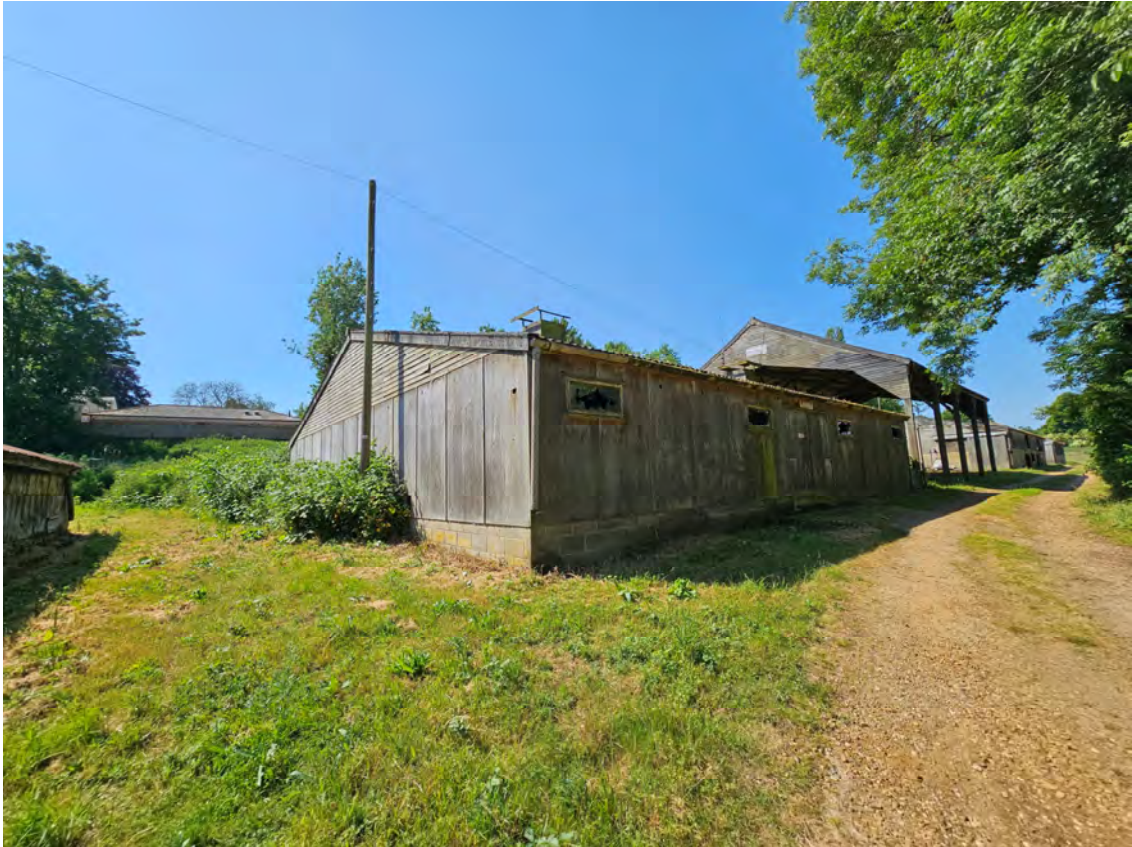
Photograph 6: Timber clad pig shed south of track (Paul Frost).
