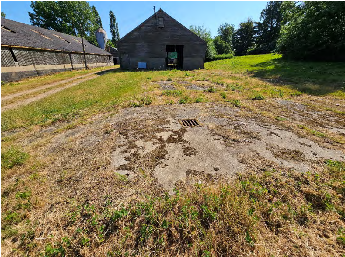
Photograph 15: View looking east at Barn A. Possible below ground slurry tank.
