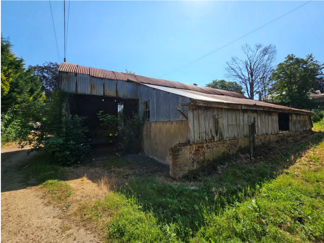
Photograph 4 : Dutch style corrugated tin clad barn south of the track.
