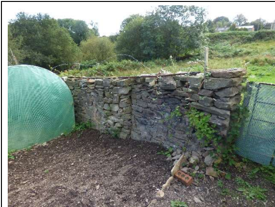
Photo 7: A (largely) dry-stone wall at the western boundary is likely to provide refuge for reptiles.
