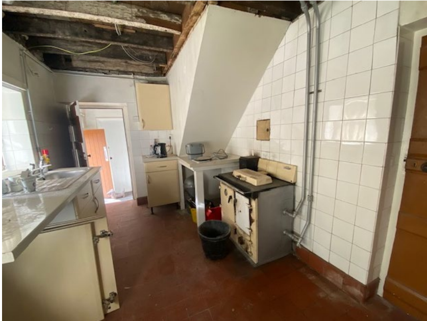
Inside ground floor of house
