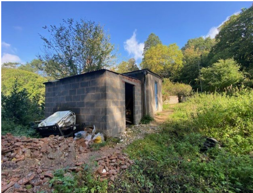
Outbuilding viewed from south-east
