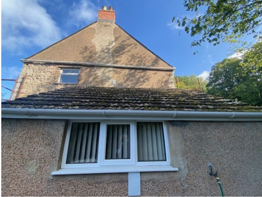
Southern gable end – no gaps on lean-to or adjacent main building
