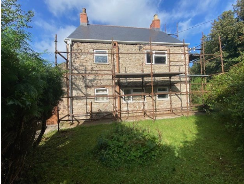
East facing elevation of house and adjacent lawn
