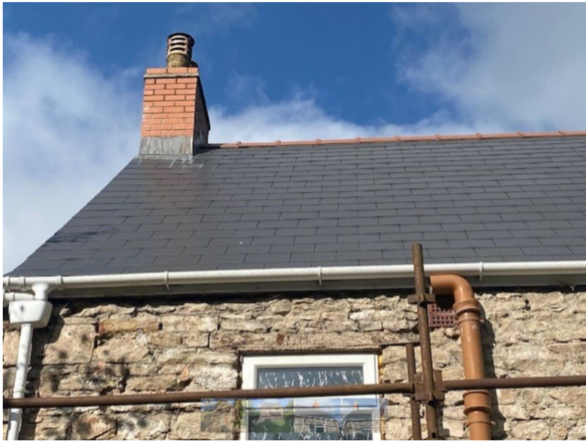
Tight fitting recent roof – east elevation
