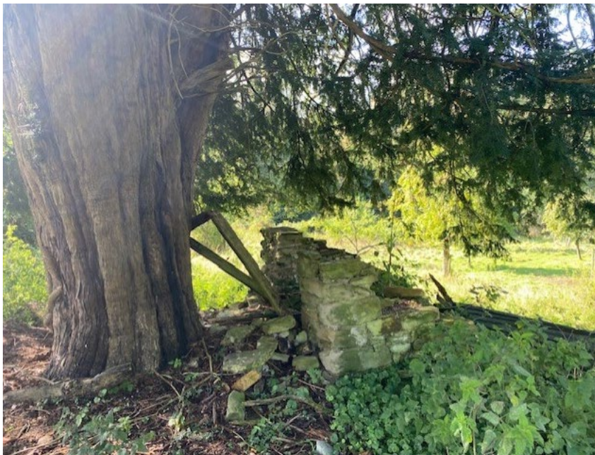
Yew tree and collapsed stone shed at south-west corner of site
