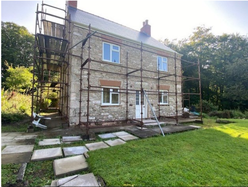
West facing elevation and adjacent lawn
