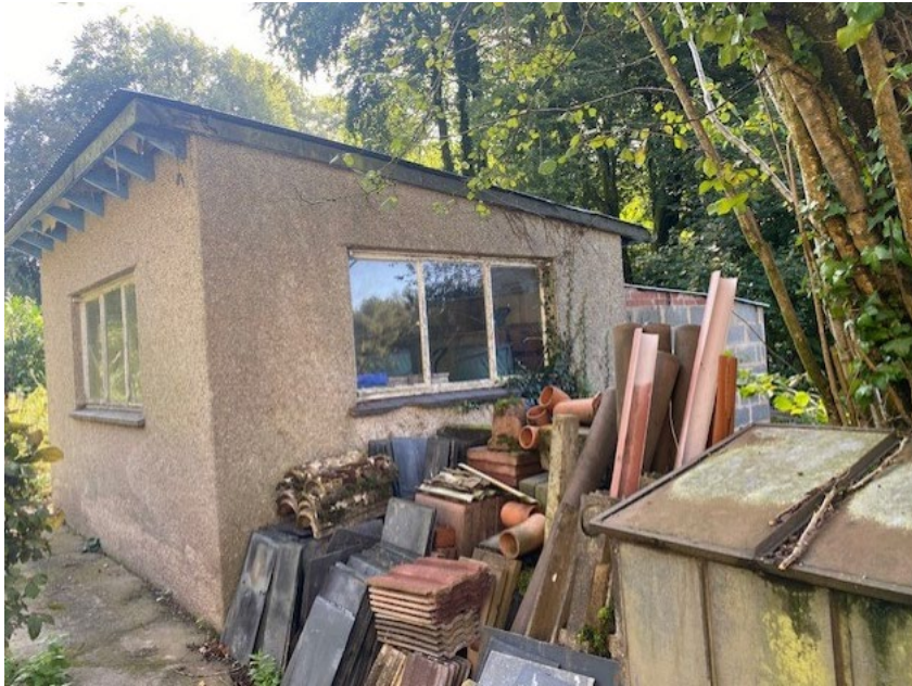
Outbuilding viewed from north-east with recently stored items
