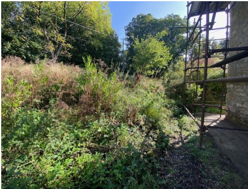
Overgrown garden bed at north gable end of house
