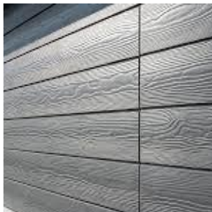
Building Grey Horizontal Shiplap Boards
