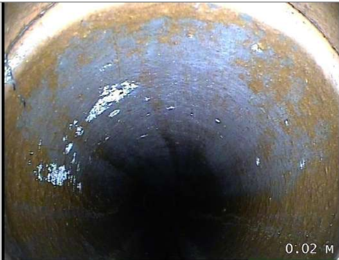
Start node type, manhole, reference FWMH1
