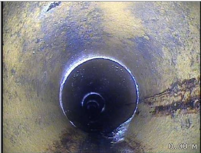
Start node type, manhole, reference FWMH4
