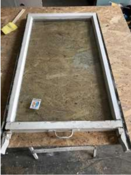
4. Double glazed unit installed and looking at the sash internally
