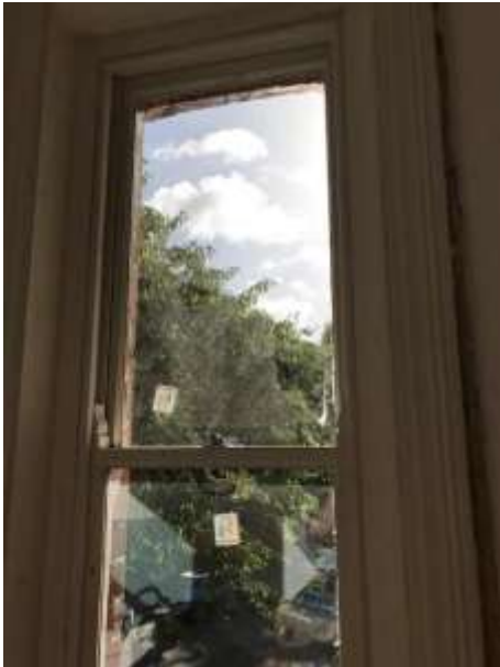
5. Double glazed unit installed and looking at the sash internally
