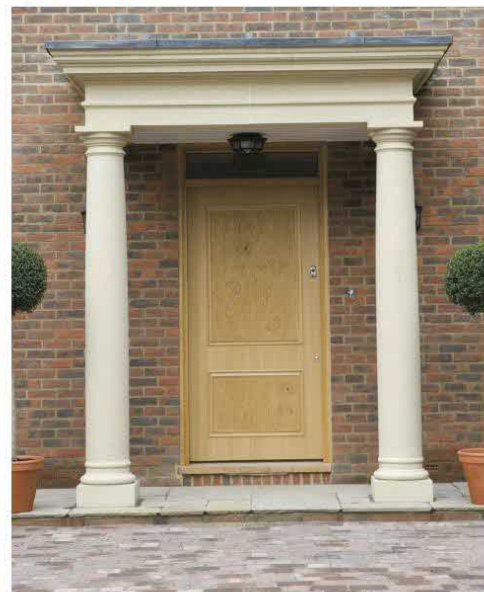
Stone Portico and detailing
