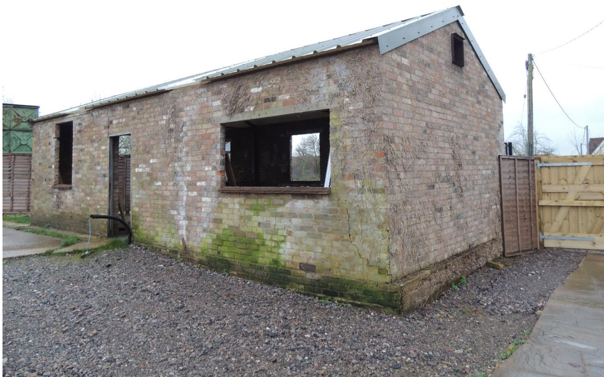
Photo 1: South-eastern (gabled) and south-western elevations
