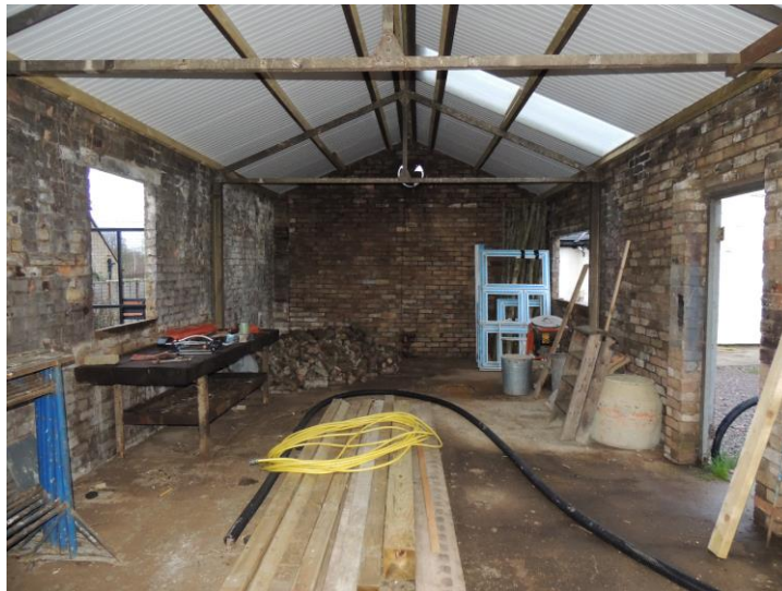
Photo 6: Looking NW-SE in the building
