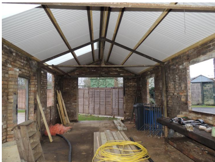
Photo 7: Looking SE-NW in the building
