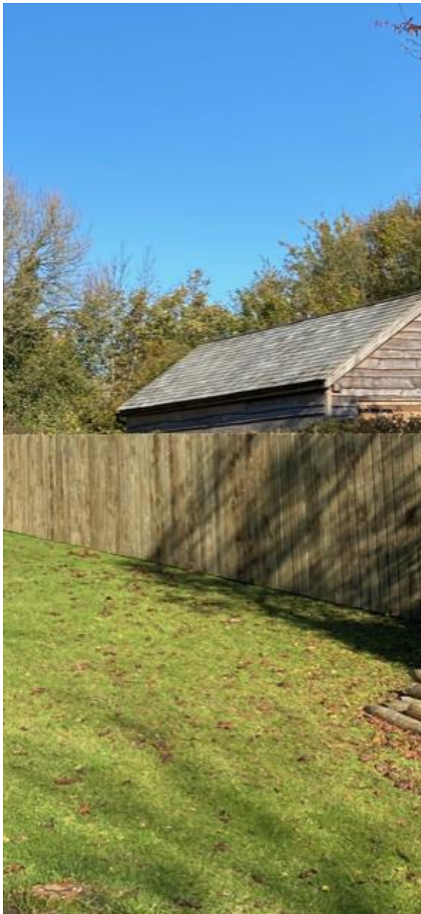
Image of vertical composite boards on galvanised steel posts to eastern side
