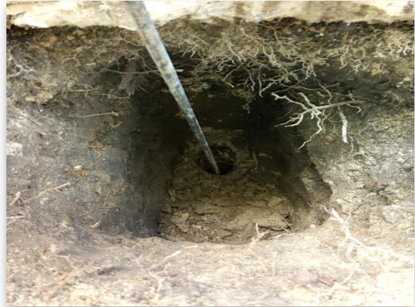
Fig 1.2: Trial Hole 1 Footing
