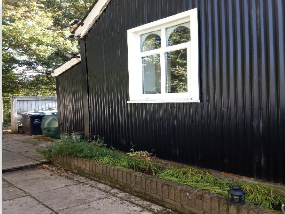
Fig 1.1: Trial Hole 1 Location
