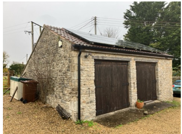
Figure 2 - Application Building Viewed From Southwest
