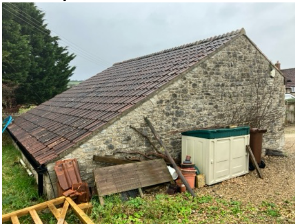
Figure 3 - Application Building Viewed Northwest
