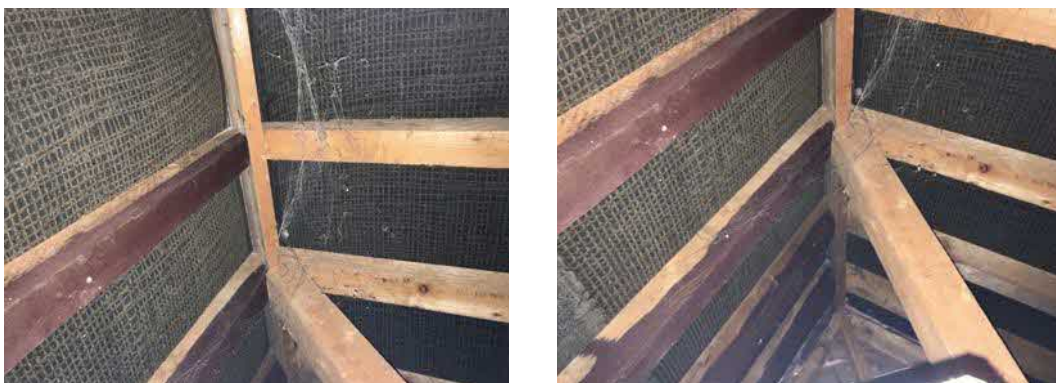
Figs. 9 & 10 Roof void of extension
