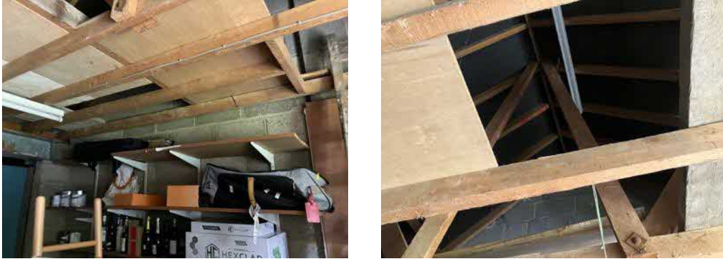
Figs. 17 & 18 Roof spare of enclosed room
