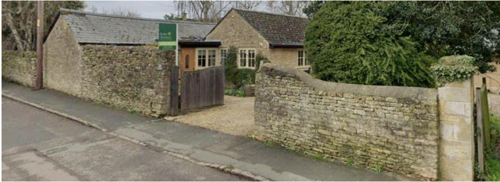
Photo 2: Detached bungalow opposite the site, set back with large shingle driveway and featuring high limestone boundary walls.
