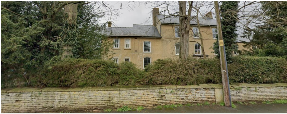
Photo 3: On the opposite side of the road from the site, next to the above property – a three and two storey building with rendered walls and a low limestone boundary wall to the front.
