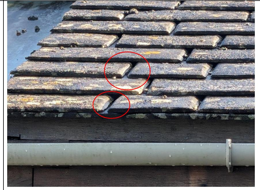
A photograph showing a section of a roof with dark stone tiles. Two red circles highlight specific areas: one on the left pointing to a gap between the tiles, and another on the right pointing to a larger area where the tiles overlap. |
