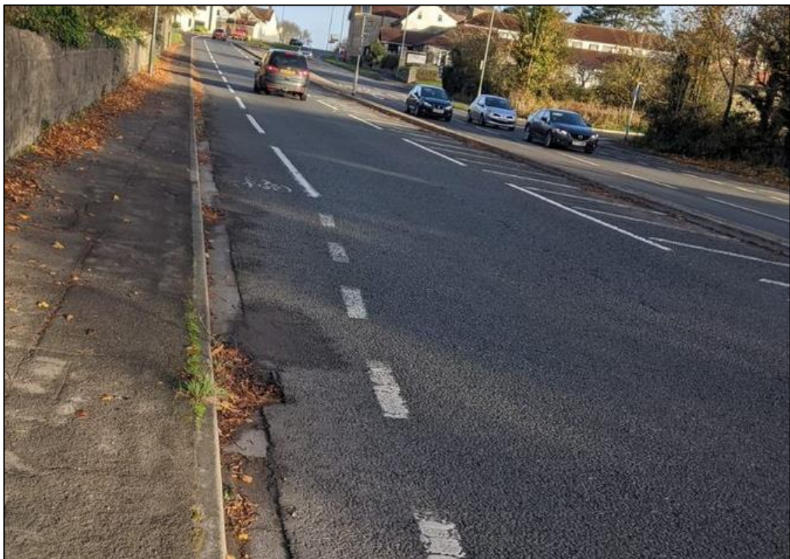
Photograph 2.7 – A38 Gloucester Road northbound on carriageway cycle lane
