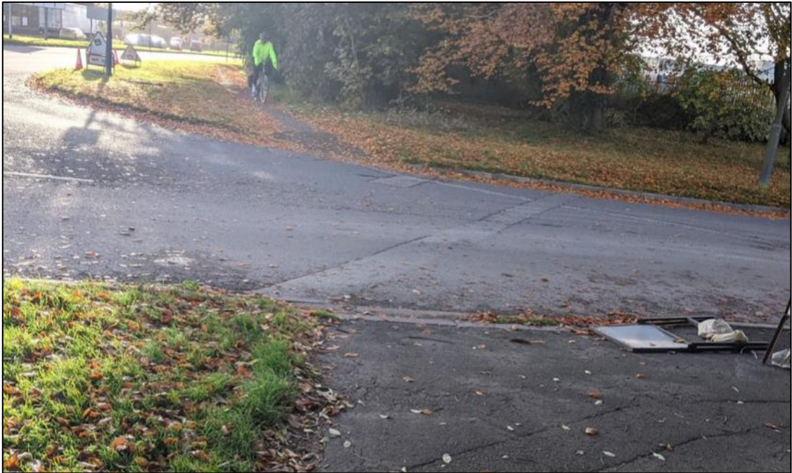
Photograph 2.4 – Existing dropped kerb crossing at the junction of Gloucester Road and A38 Gloucester Road
