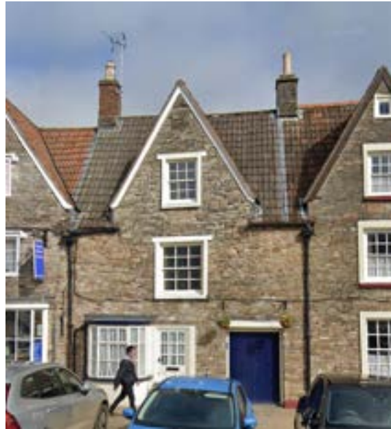
Photograph 01 – View of the principal southern elevation.
