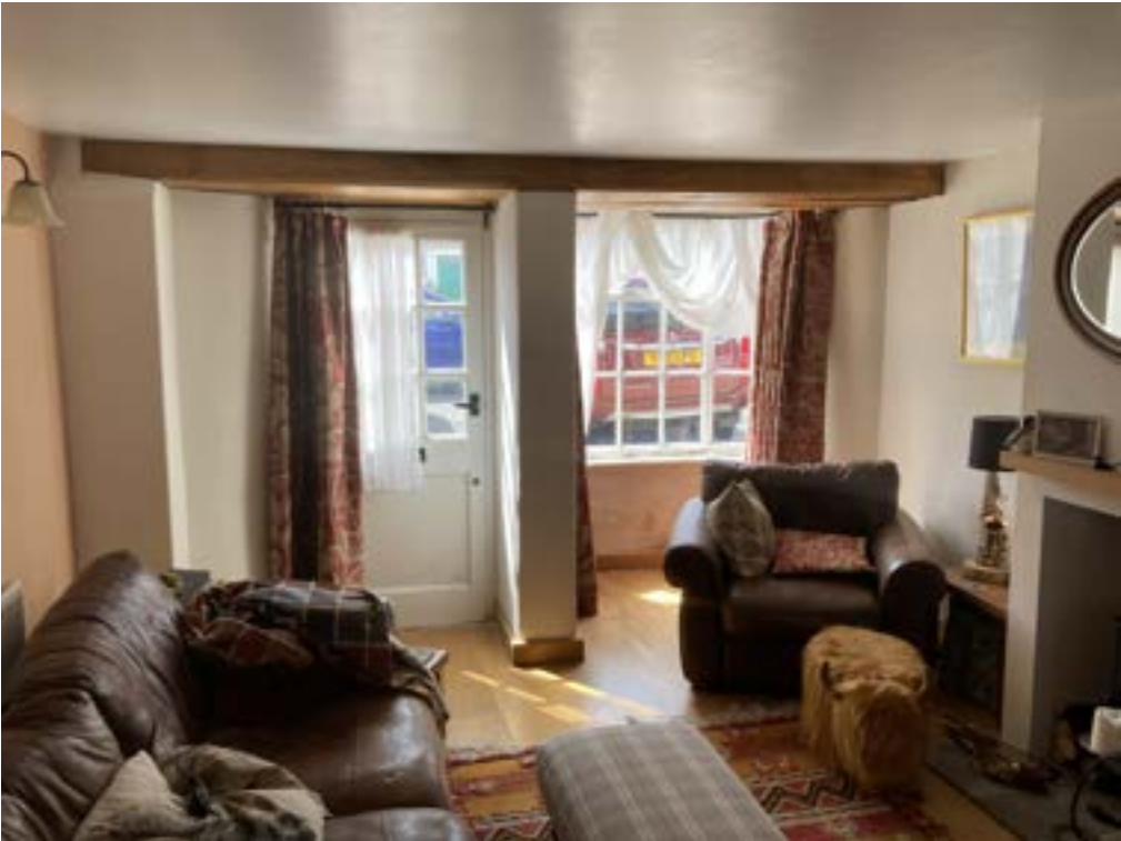
Photograph 03 – Internal view of the bay window and door to which this application relates.
