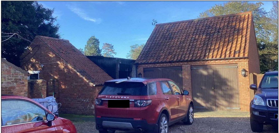
Photograph 1.3.2: View of the south elevations of Building 1 (the workshop) on the right (east) and Building 2 (the storage shed) to the left (west).
