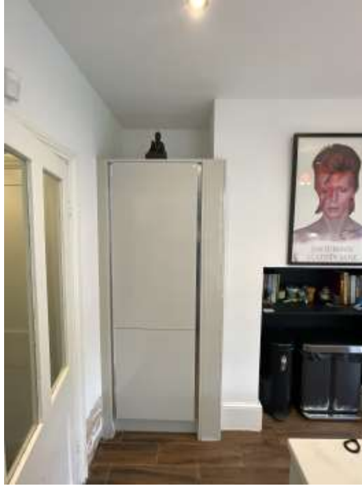
Photograph 3 – Kitchen chimney breast; Left hand side
